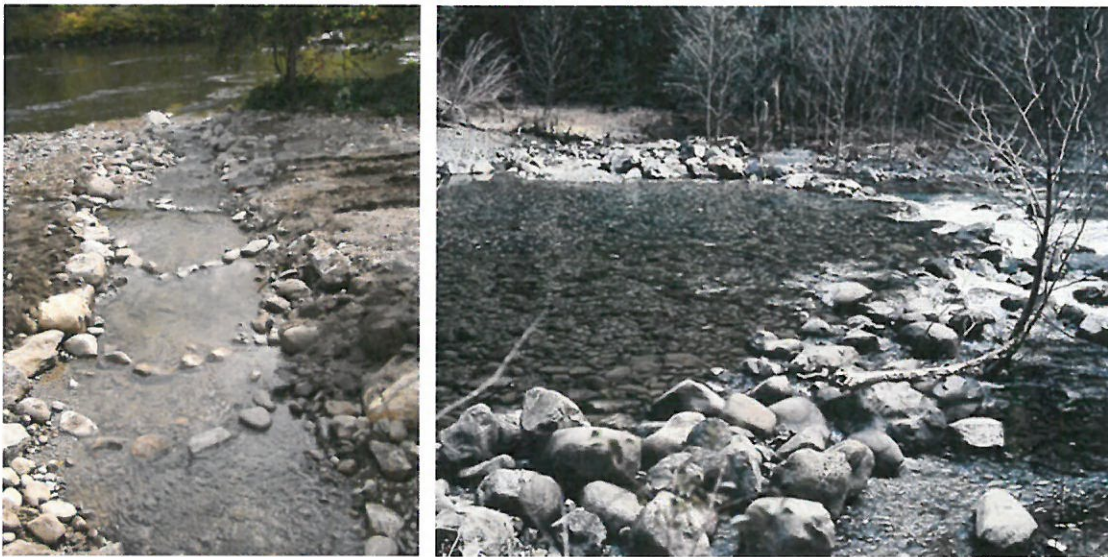
Figure 2. Examples of local cobble used to constrict flow and provide improved fish passage conditions in both small and moderate sized streams. Left picture: Spruce Brook, Connecticut, Department of Energy and Environmental Protection. Right picture: Hurdygurdy Creek, California, USDA.
