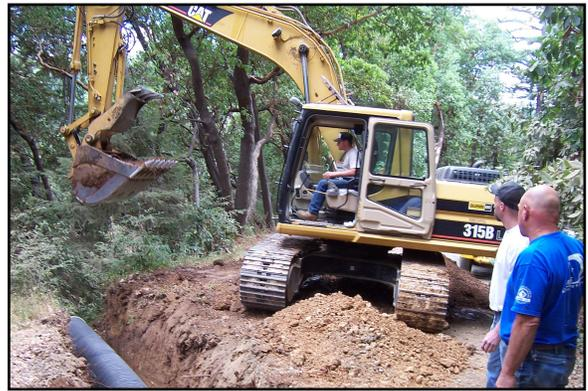
Workers install a properly sized culvert to capture water emanating from steep slopes above this rural road and direct it to a location protected from erosion.
