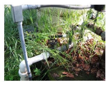
Overgrowth of vegetation near your well may lead to root damage of the casing, creating a conduit for possible well water contamination.
