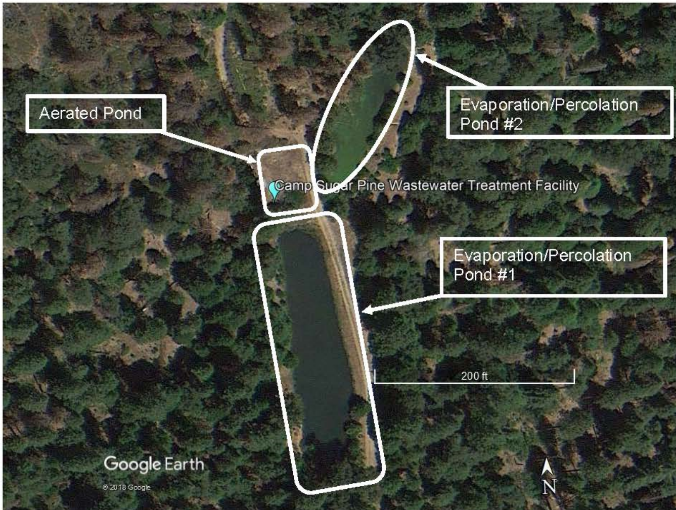
ATTACHMENT B – WASTEWATER PONDS MAP NOTICE OF APPLICABILITY 2014-0153-DWQ-R5340 FOR SUGAR PINE CHRISTIAN CAMPS CAMP SUGAR PINE WASTEWATER TREATMENT SYSTEM MADERA COUNTY
