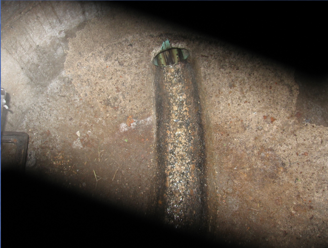
Sewer corrosion below a coffee shop
