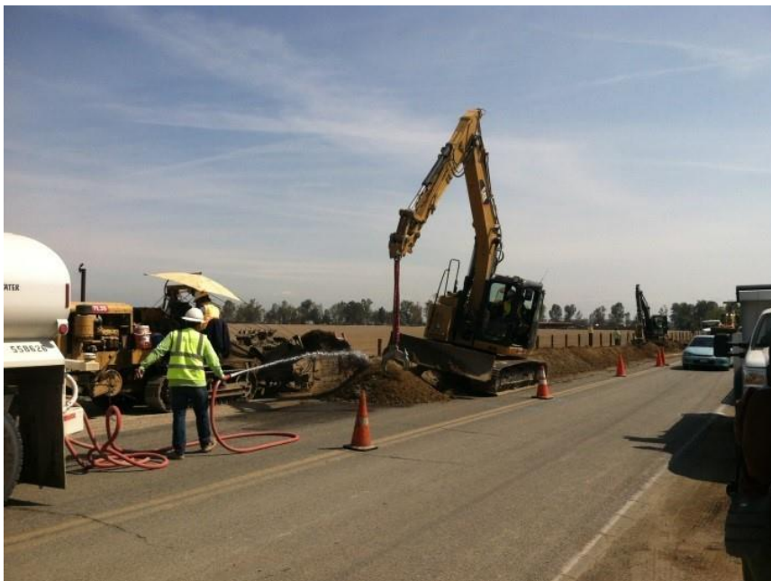
Photo 1 Construction of intertie to California Water Services.
