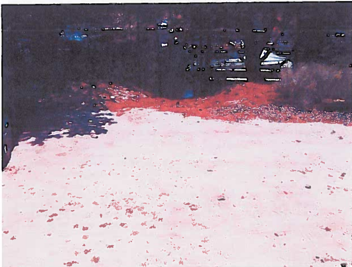
Picture 1: The parking lot is composed of exposed loose dirt and a small amount of gravel on the edges. The depression in the photo is a gangway to the marina slips below. There is no berm protecting this area from concentrated flow down along the gangway causing erosion.
