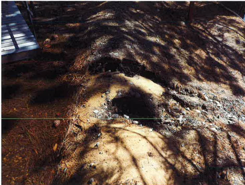
April 20, 2017. Eroded berm at STA WEST 2+40 looking east showing signs where water surface elevation in swale exceeded the design water surface elevation causing erosion.
