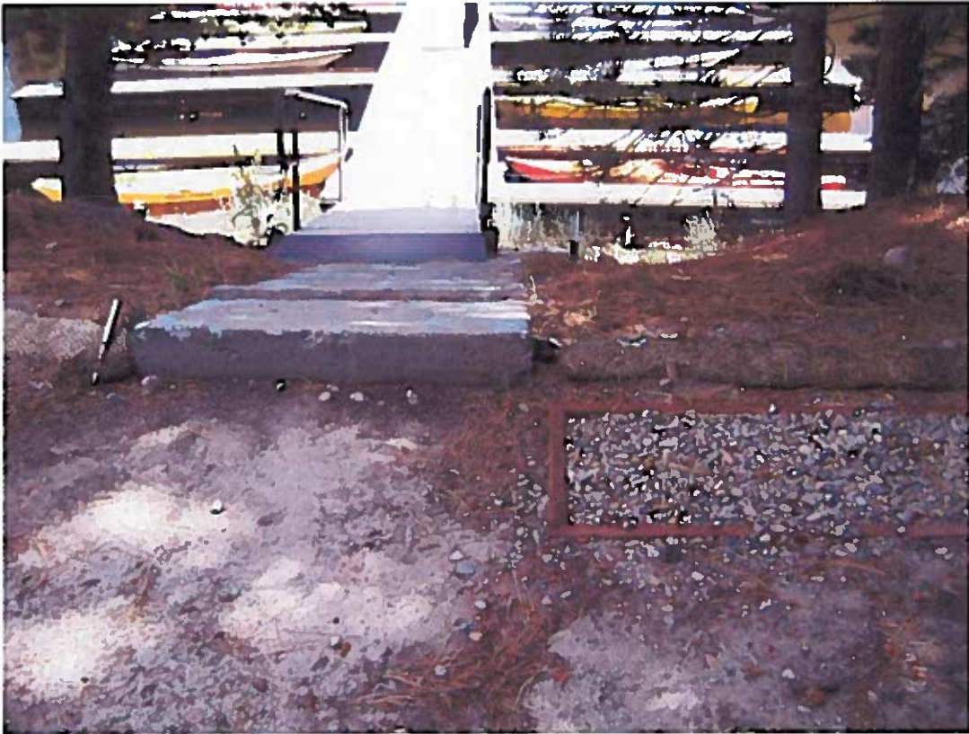
Photograph 07 - First ramp west of office, facing south. A gap exists between the concrete section of the ramp walkway and the fiber roll to the right (west) of the ramp. Runoff that bypasses the drainage ditch will flow through this area and into the marina.
