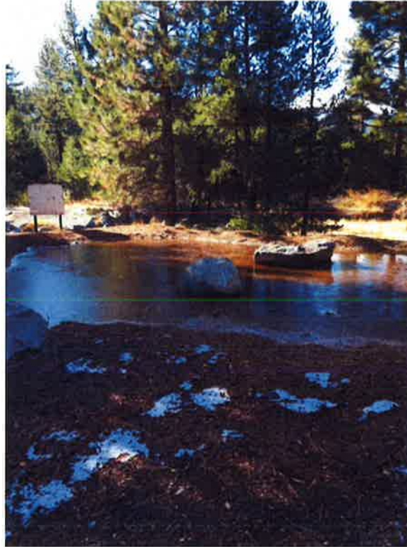
November 1, 2016. Basin and berm at STA WEST 4+00 following precipitation.
