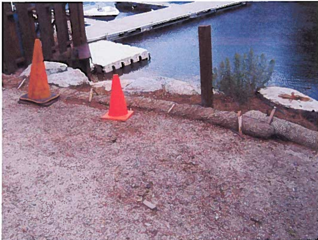
Photograph 06 - BMP joint is not J-hooked, and the fiber roll section by the pylons has been flattened. This area is by marina office, facing southeast
