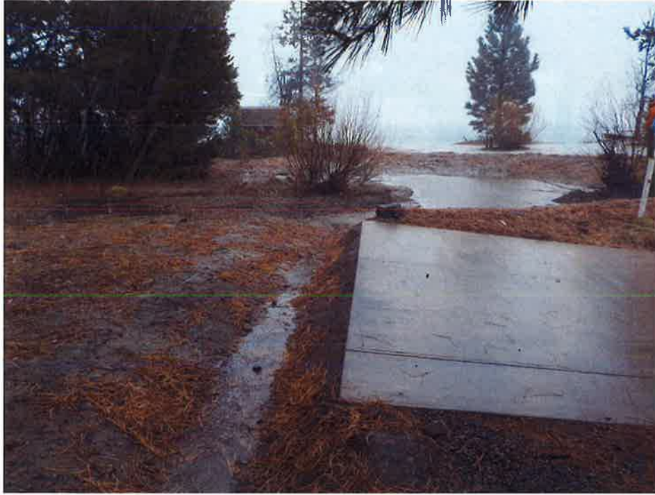
December 10, 2015. Swale and basin looking east at STA EAST 2+00 following precipitation.
