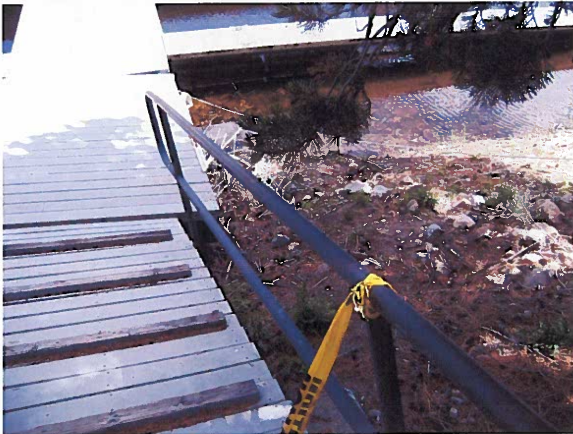
Photo 14 – From same location as Photograph No. 13, but looking on the west side of the second ramp west of office.
