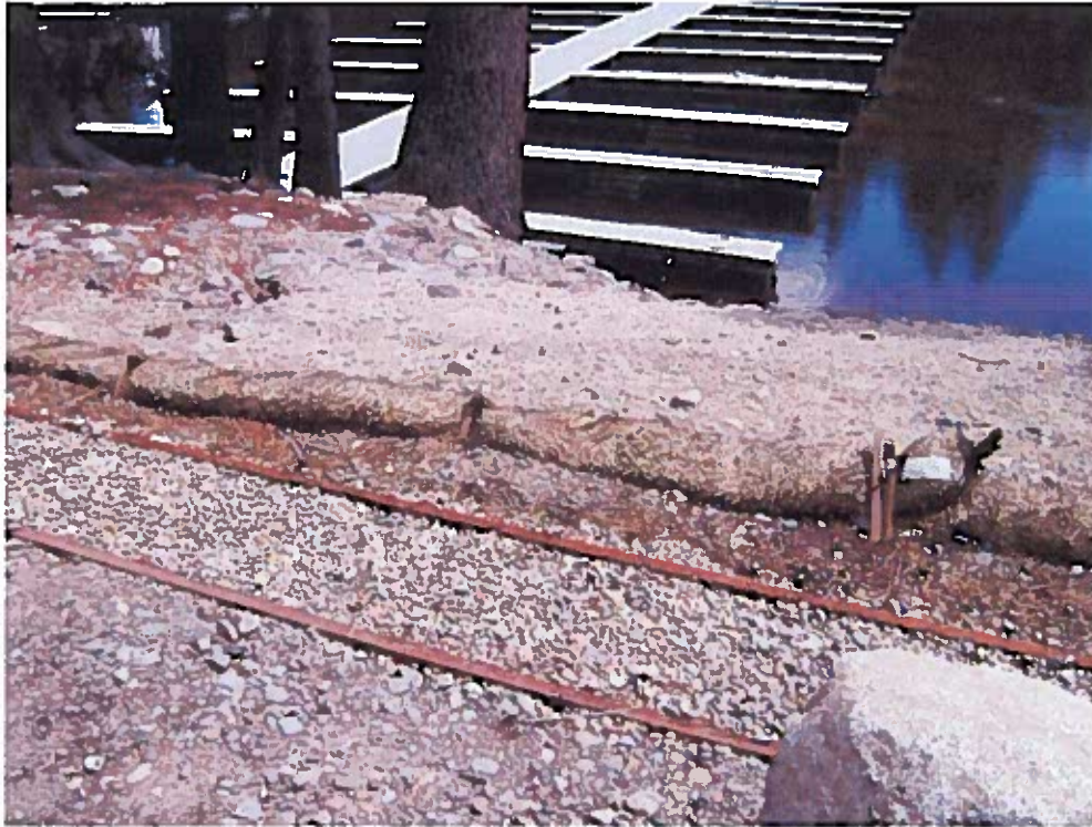
Photograph 15 - About 20 feet west of 2nd ramp west from office, looking south-southeast. The fiber roll has been degraded degraded and flattened.
