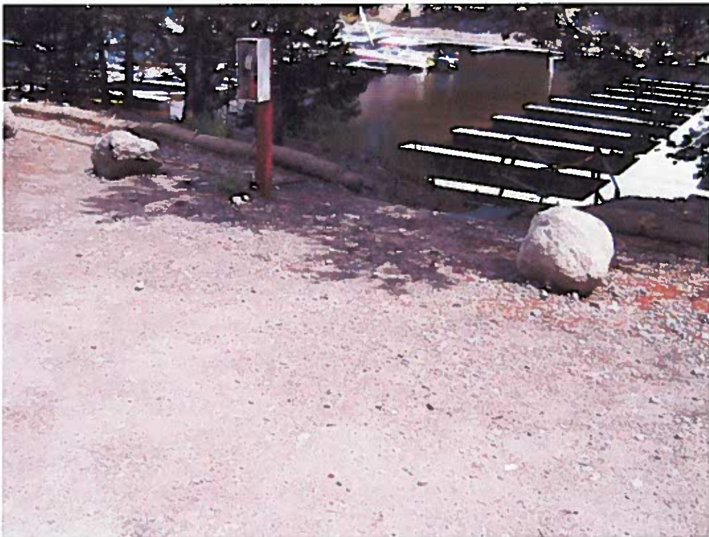
Photograph 08 - Second ramp west of office, facing southeast. Fiber rolls do not prevent runoff from going down ramp and into marina.
