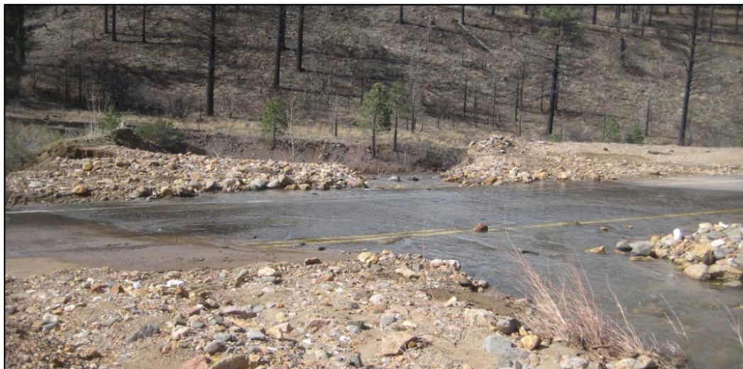
Erosion damage from flows bypassing clogged culvert and overflowing over State Highway 4. The East Fork
