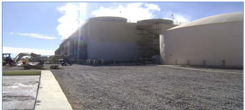
Figure 1 Photo showing HDPP cooling towers using extracted water for cooling purposes. Visible steam is released to the atmosphere.
