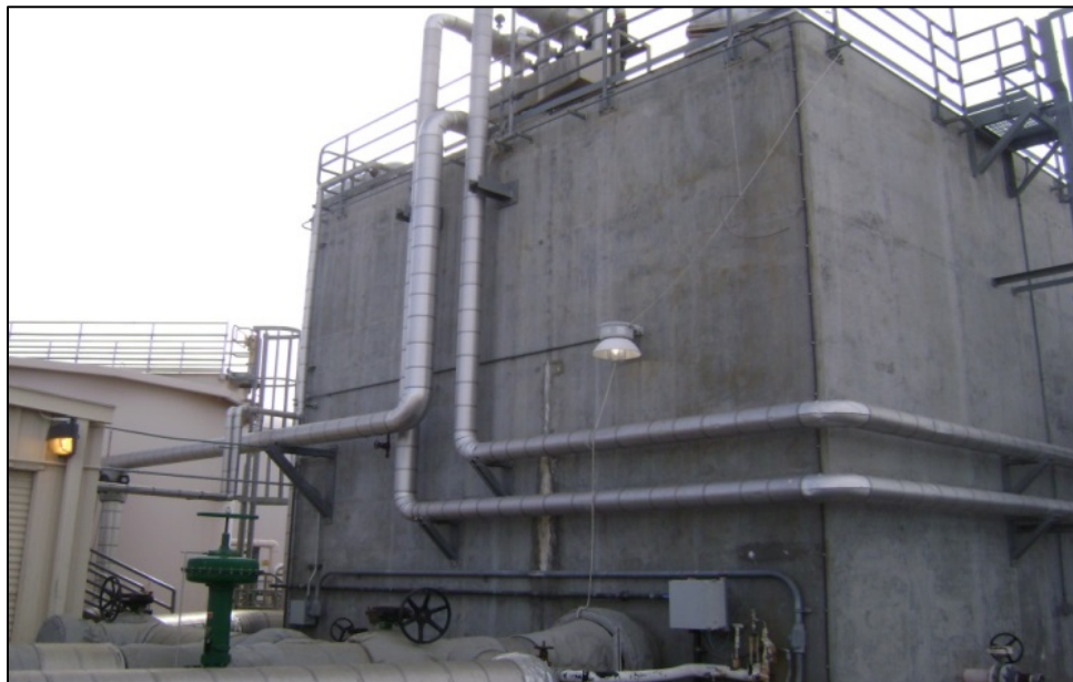
Photo showing a filtration structure at the HDPP as part of the water treatment process prior to injecting treated water into the Mojave River Regional Aquifer.
