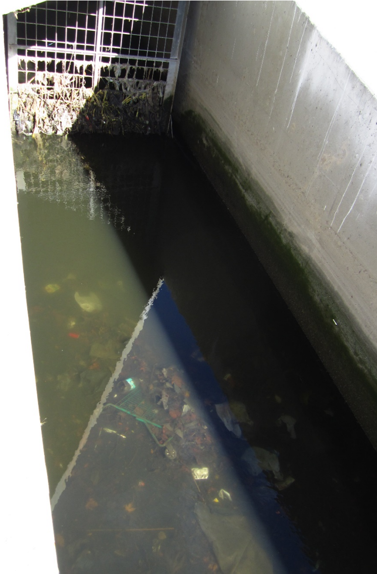
Figure 5 Storm drain in Ballona Creek clogged with plastic bags and trash, including a shopping cart. December 14, 2013.
