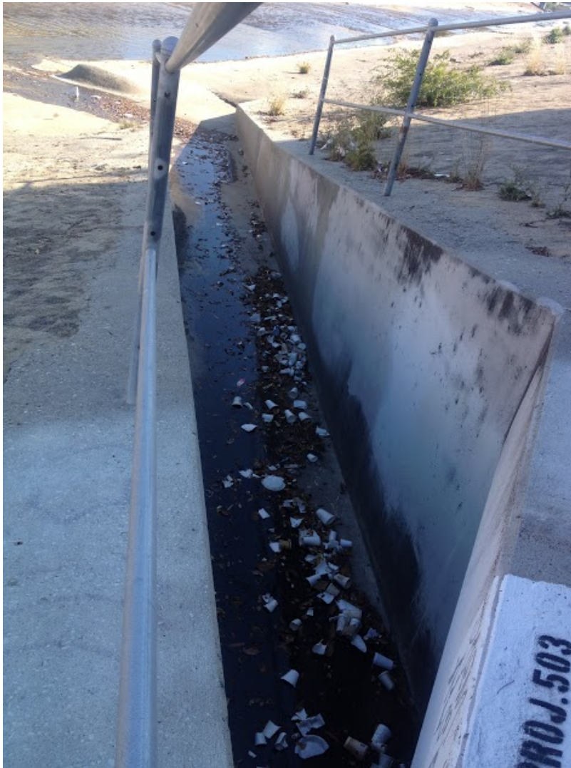
Figure 1 Foamed plastic and other trash flowing from a storm drain into Ballona Creek. May 15, 2015.
