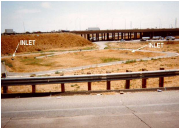
Figure 5-11 Regional Infiltration Basin
