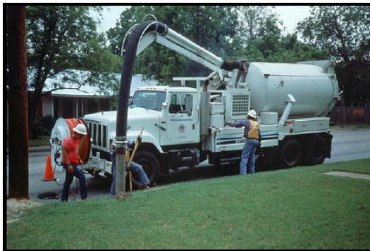
Figure 5-15 Catch Basin cleaning
