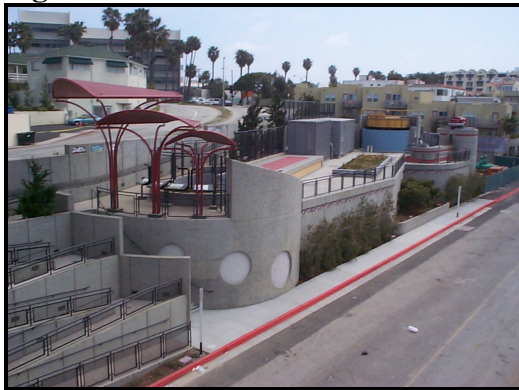
Figure 5-10 Santa Monica Urban Runoff Recycling Facility (SMURRF)
