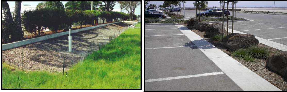
Figure 3: Infiltration Trenches (CASQA, 2003b; USEPA, 2006)
