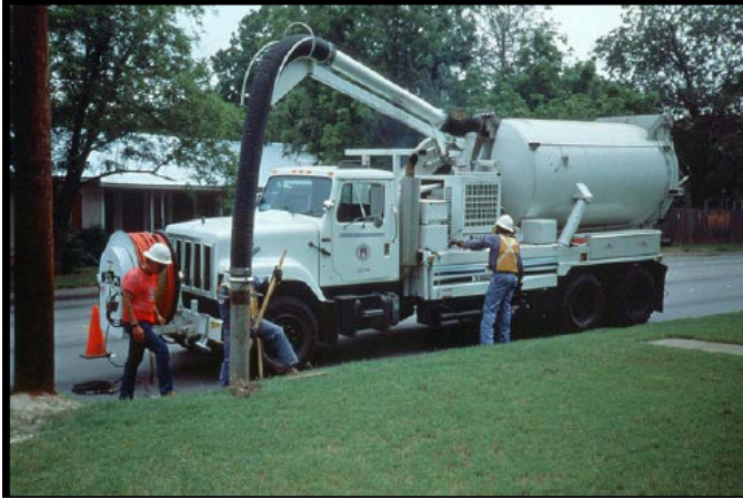
Figure 5-10: Catch Basin cleaning(Source:CASQA, 2003a)
