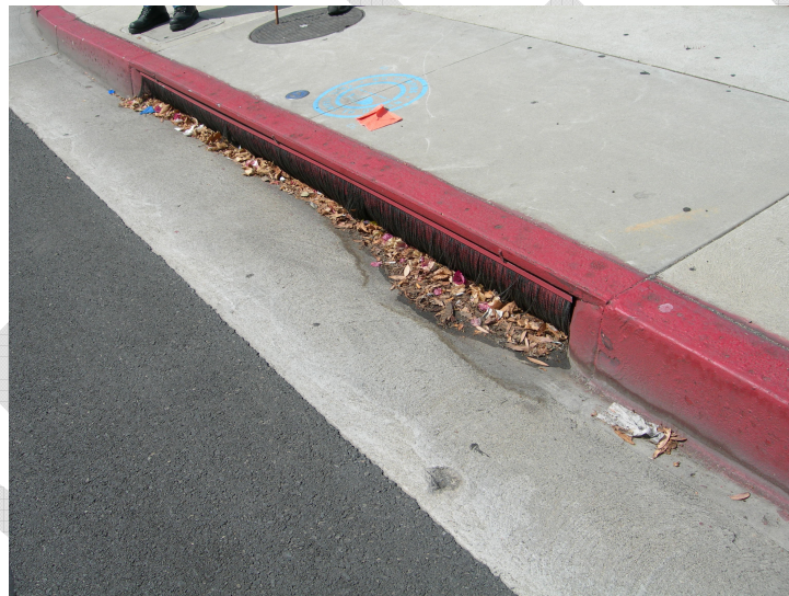
Figure 7.3-2. A catch basin brush insert with accumulated debris
