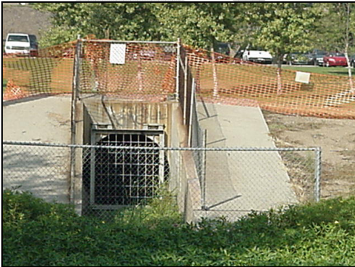
Figure 8-6. Machado Lake trash screen. Machado Lake is in the Ken Malloy Harbor Regional Park, in the Dominguez Channel Watershed.
