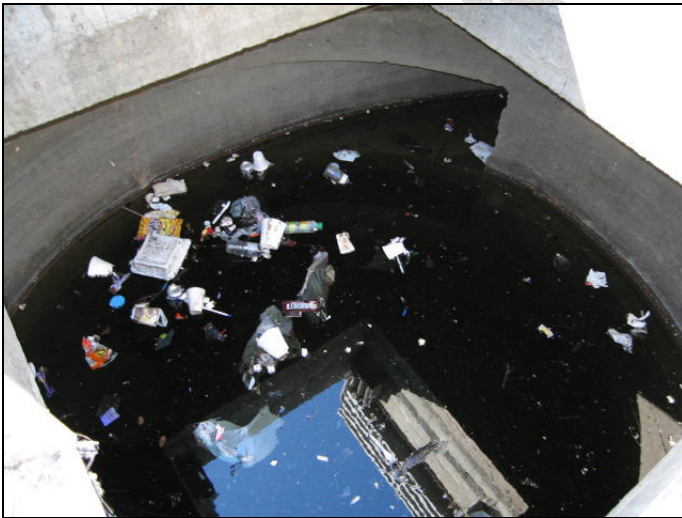
Figure 8-3. Example of Inline CDS unit, Pico-Kenter drain in the City of Santa Monica
