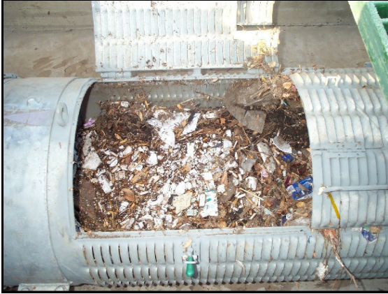
Figure 8-6. Caltrans GSRD Unit Linear Radial GSRD (LR1 I-10) off the I-10 Freeway at Rosemead
