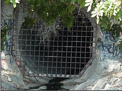
Figure 8-7. Machado Lake trash screen. Machado Lake is in the Ken Malloy Harbor Regional Park, in the Dominguez Channel Watershed.
