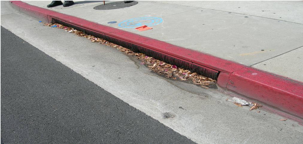
Figures 6-5 Brush installed over the catch basin opening.
