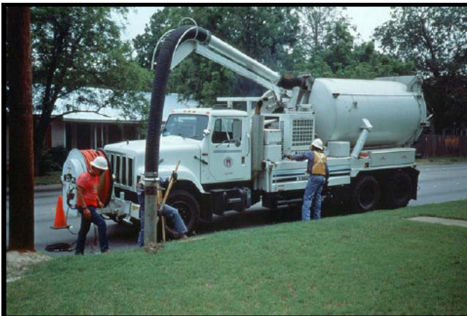
Figure 6-12: Catch Basin cleaning (Source: CASQA, 2003a)
