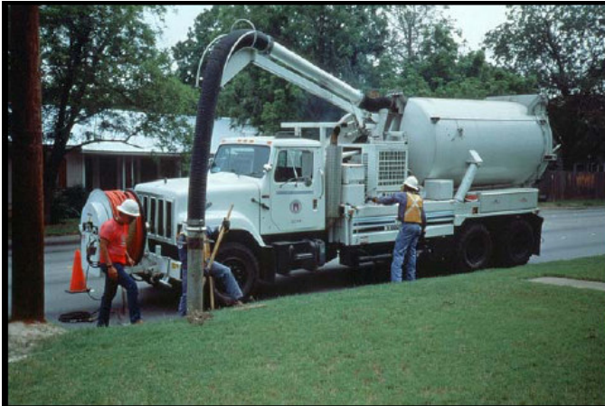
Figure 5-13: Catch Basin cleaning (Source: CASQA, 2003a)
