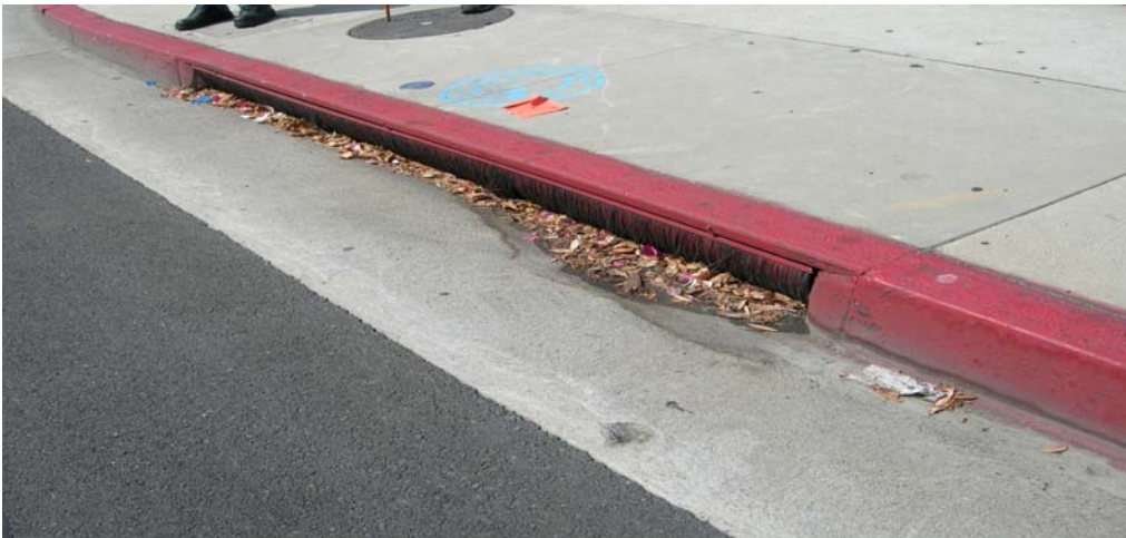
Figures 5-5 Brush installed over the catch basin opening.
