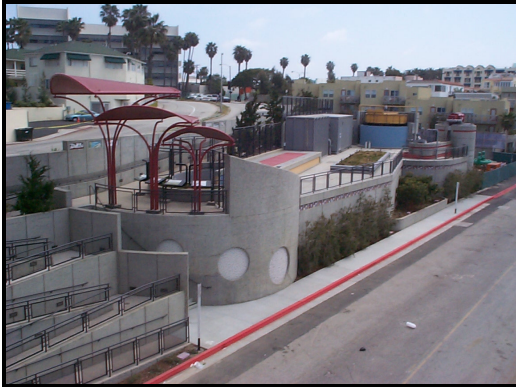
Figure 5.9. Santa Monica Urban Runoff Recycling Facility (SMURRF)
