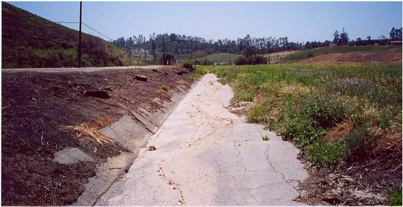
Proposed re-lining of downstream eroded area.
