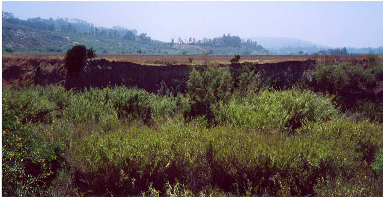
Proposed repair included laying back the slope, planting native grasses on the slope and willows and mule fat at the toe.
