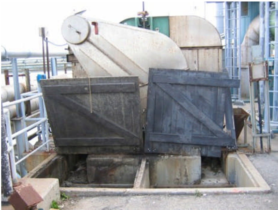
Figure B4-3. Units 3&4 (8-10) traveling screens sump collection area. The Unit 5&6 sumps are similar.
