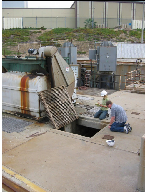
Figure B4-1. Collection sump next to traveling screens, SGS Units 1-2
