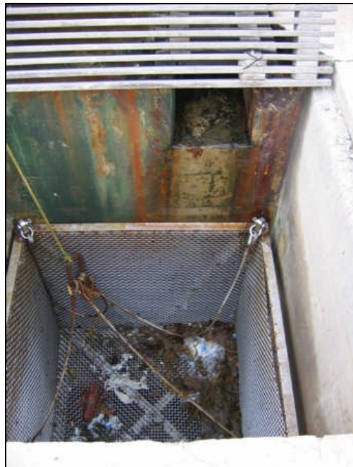
Figure B4-2. Collection basket at SGS Unit 3.
