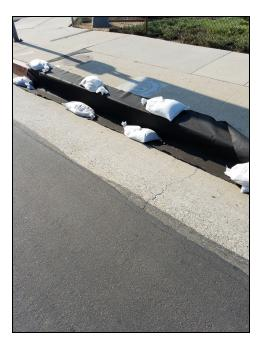
Figure 5. Catch basins along the study routes were covered to prevent trash from being swept into them.
