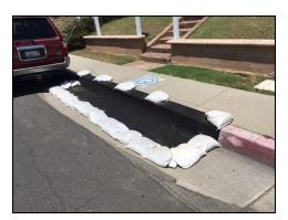
Figure 8. Catch basins along the study routes were covered to prevent trash from being swept into them.
