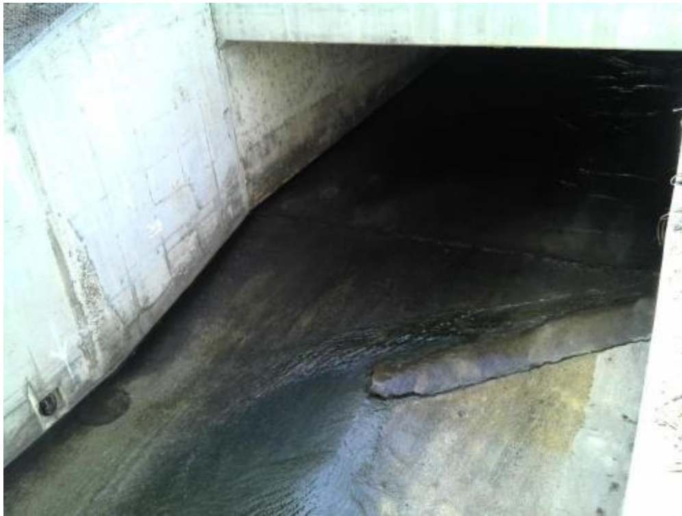
MCC_VAL Ground-Level View
