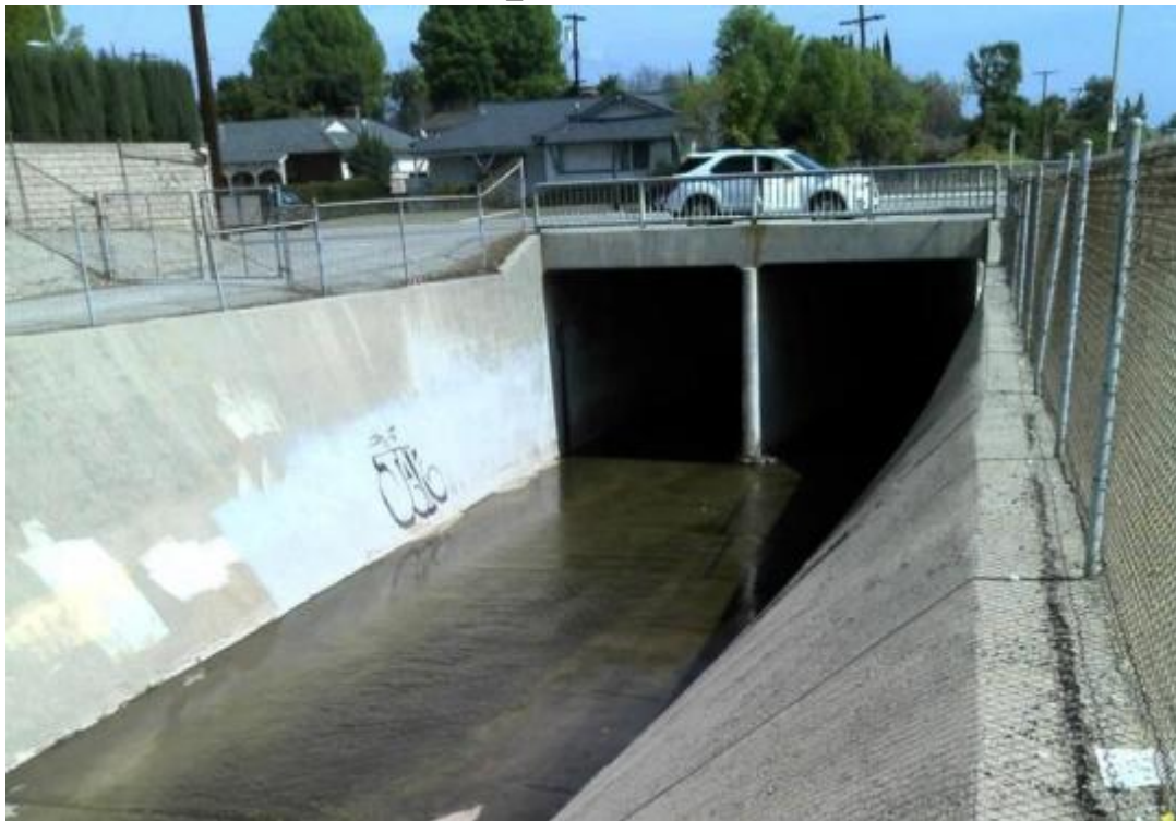
BEL_FAL Ground-Level View
