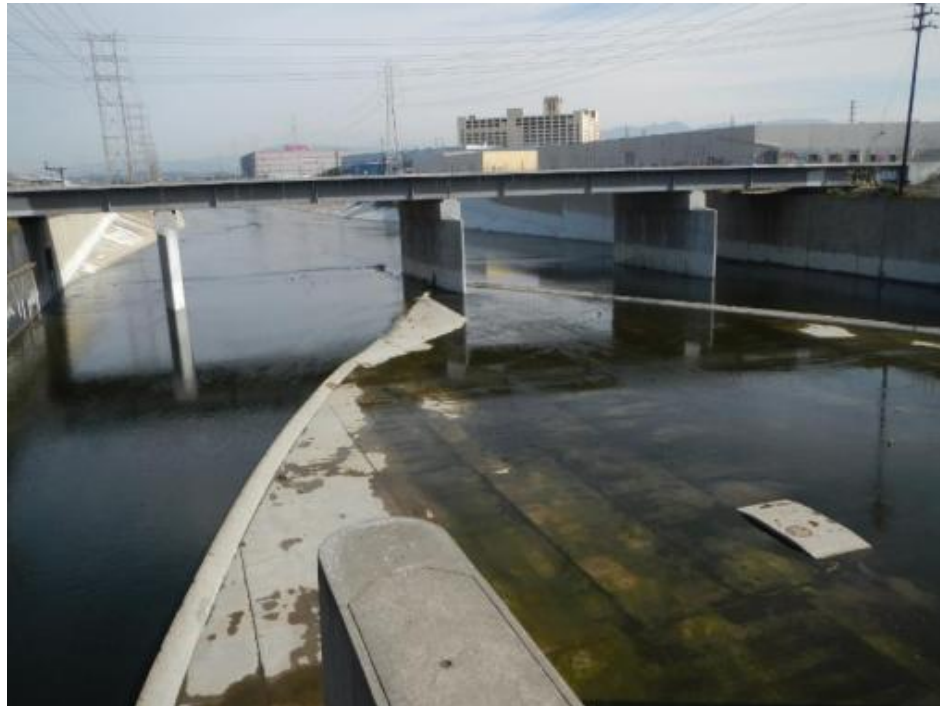
LAR_02_WAS Ground-Level View
