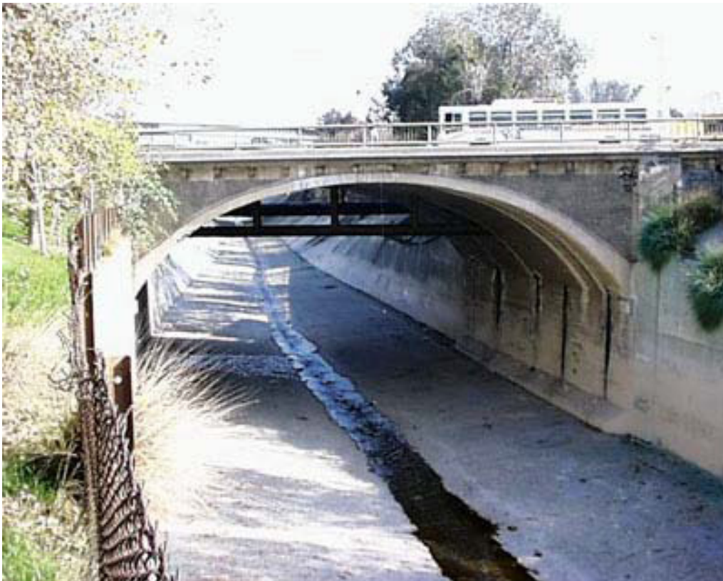
AS_SAN Ground-Level View
