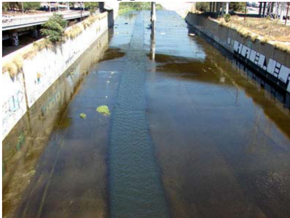
LAR_03_FIG Ground-Level View
