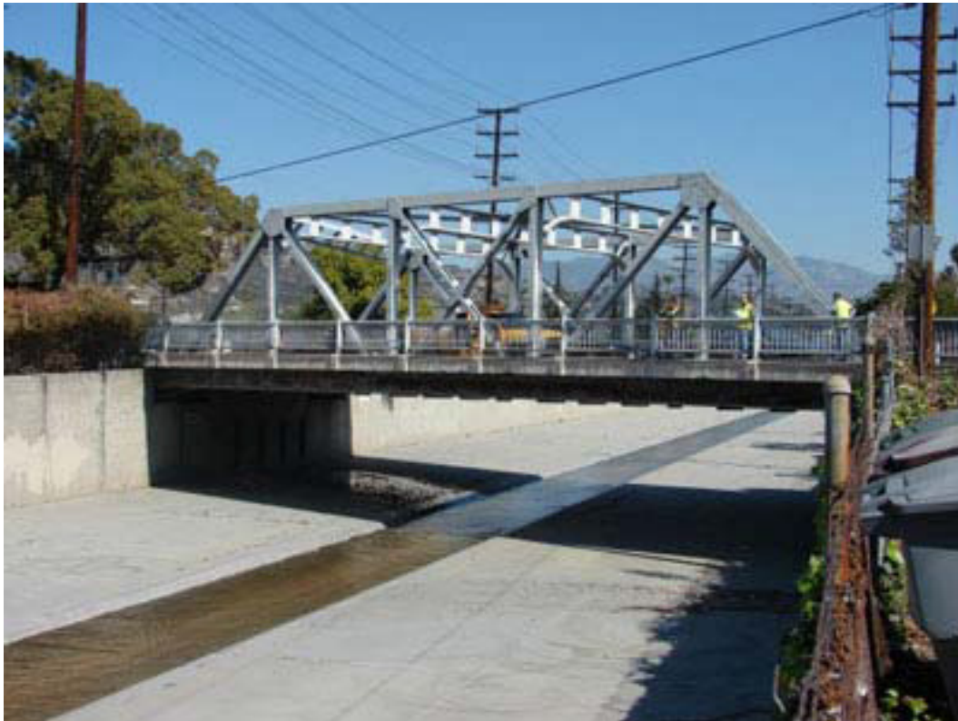
VW_CON Ground-Level View
