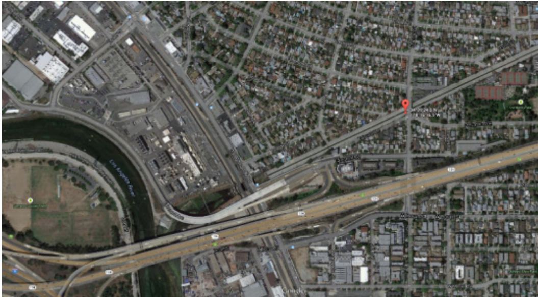
VW_CON Aerial View
