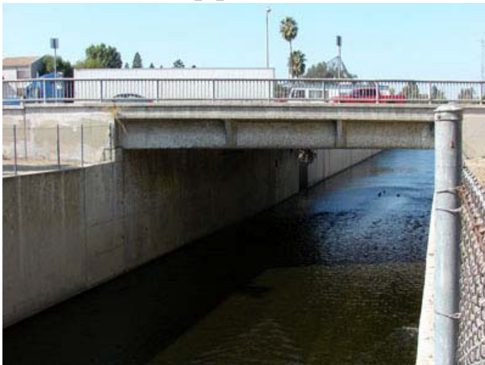
LAR_05_SEP Ground-Level View
