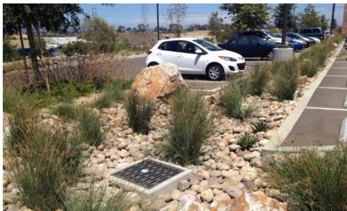
Recently constructed biofiltration in a parking lot
