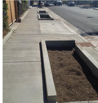
Newly constructed bioretention cells along Brandon Street
