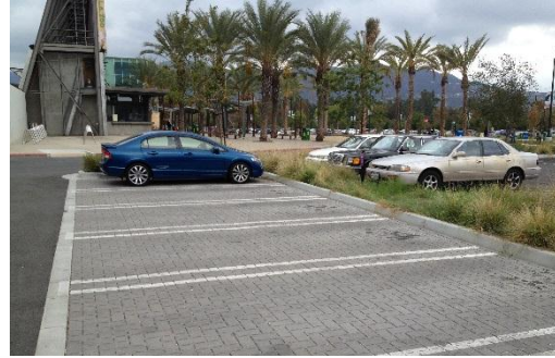
Bioretention and permeable pavement at the Los Angeles Zoological Park
