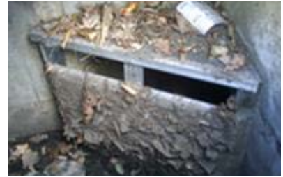
Connector Pipe Screen
