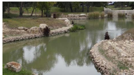
Wet Detention Pond
