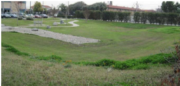
Surface Infiltration Basin
