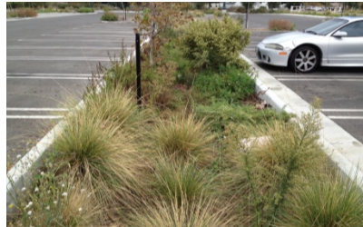
Parking Lot Biofiltration
