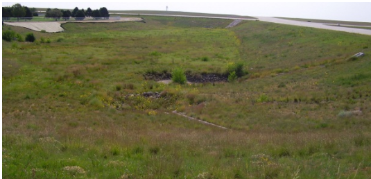
Surface Detention Basin
