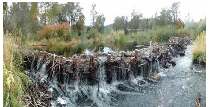
Figure 1: BDA constructed by the Scott River Watershed Council on Sugar Creek.
