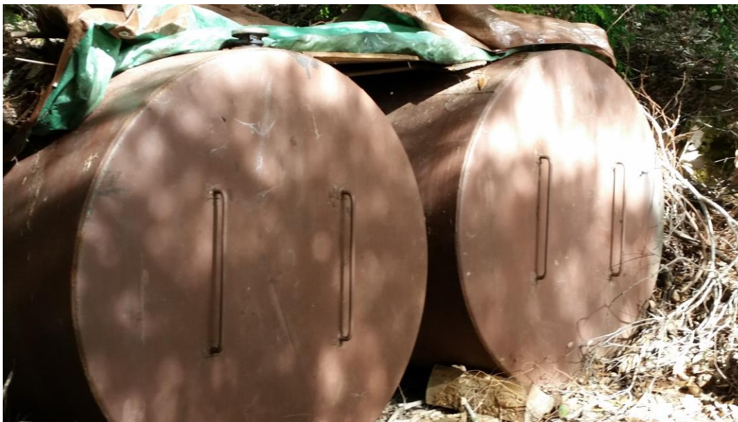
Photo 1. Two 1000-gallon AST. Tanks are located on wooden pallets. There is no visible or olfactory indications of a hazardous material spill or soil contamination.
