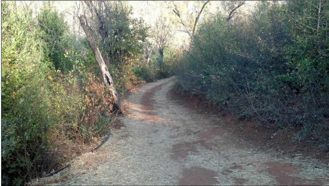
Photo 1. View of the Main Access Road through the XYZ Ranch with low cutbanks and small berm visible at the outboard edge of the road (Map 1).
