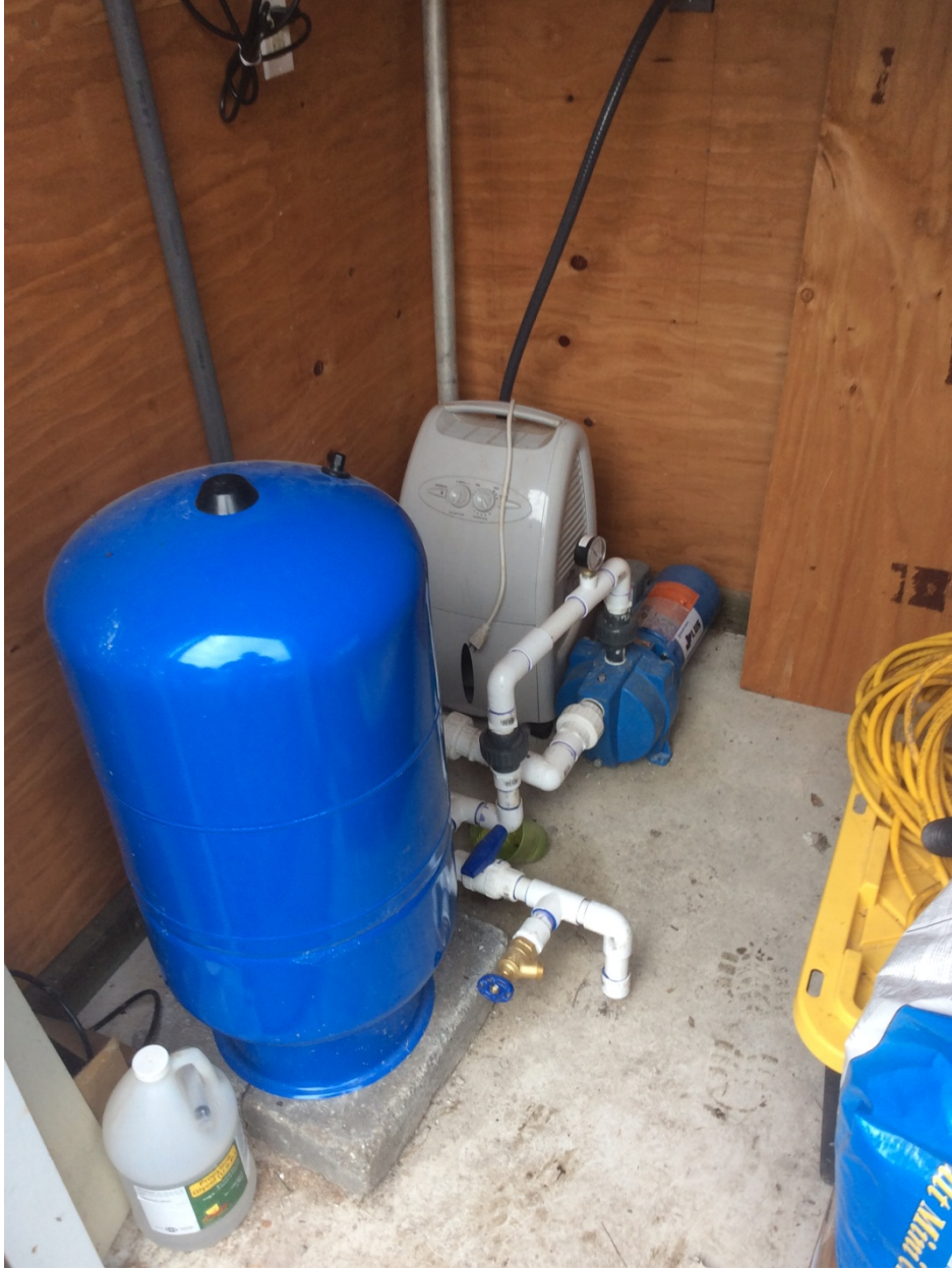
Picture 7: This photograph is of the irrigation well. Photo date 2-18-16.
