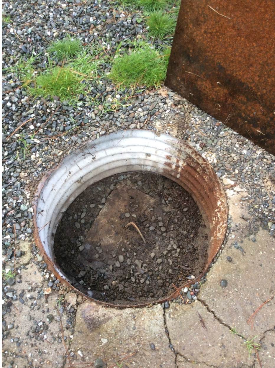
Picture 5: This photograph is of the hatch for the septic tank. Photo date 2-18-16.
