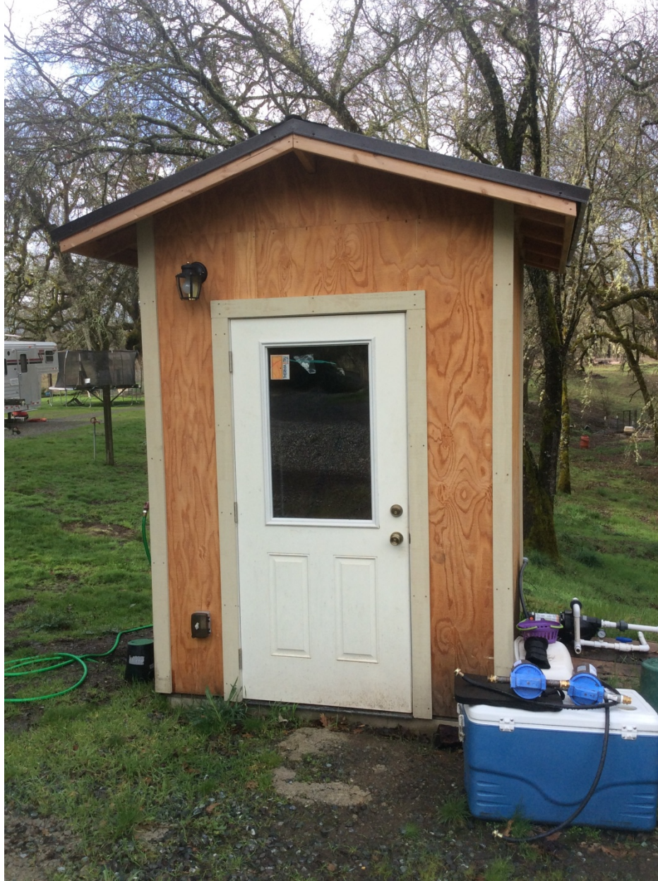
Picture 9: This photograph is of the chemical storage building facing west. Photo date 2-18-16.
