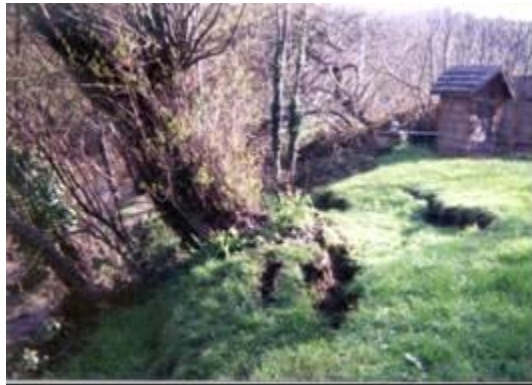
Figure 3.7 Bank slump on Upper Mainstem Elk River (Photo by Nancy Sievert, 2003).
