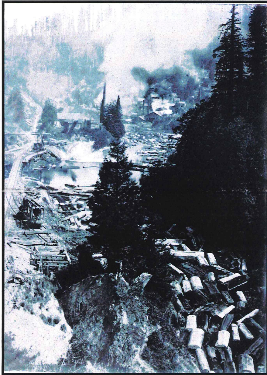
Figure 2. Looking downstream at the town of Falk in the South Fork of the Elk River circa 1900. The picture indicates at least two dam structures (from the Humboldt Room Photographs Collections).
