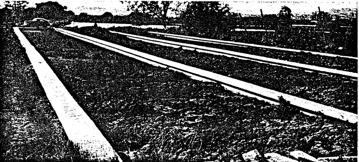
PHOTO 4 - Santa Rosa Sewer Farm showing concrete settling tanks with crust.
