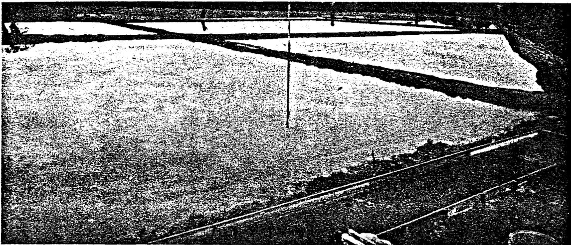
PHOTO 16 - Sebastopol Sewage Disposal Plant. Sludge drying beds and oxidation ponds. Effluent from latter to Laguna at farthest corner in right distance.
