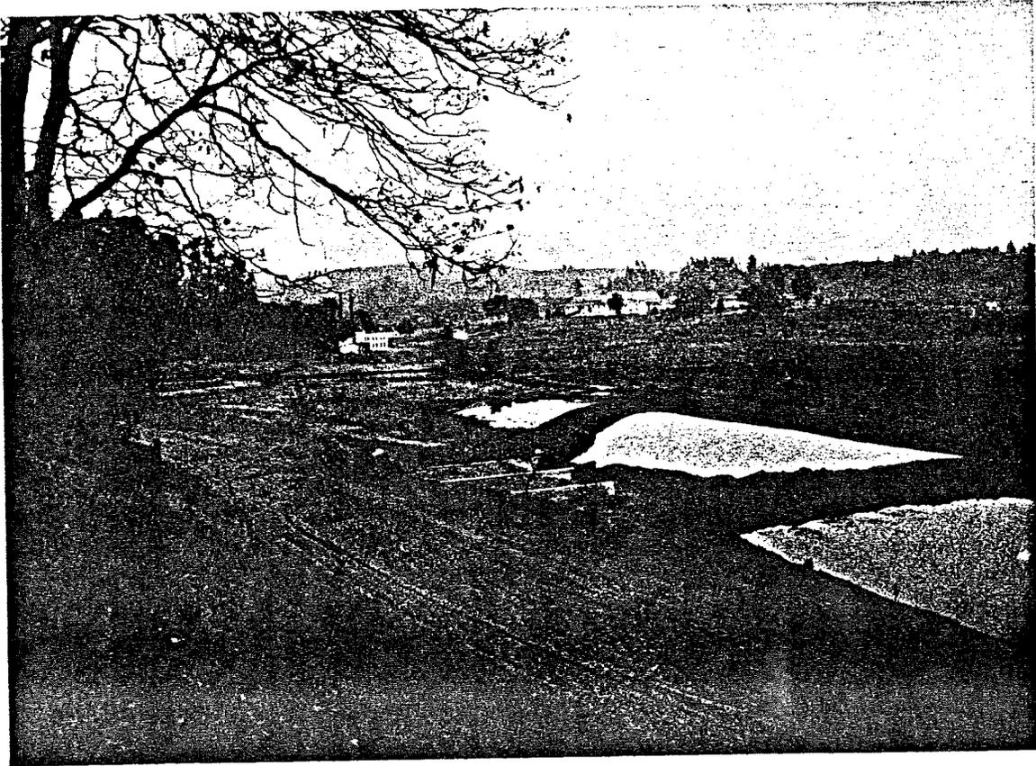
PHOTO 22 - Sonoma County Hospital showing old Dunbar filter and newly constructed oxidation basins.
