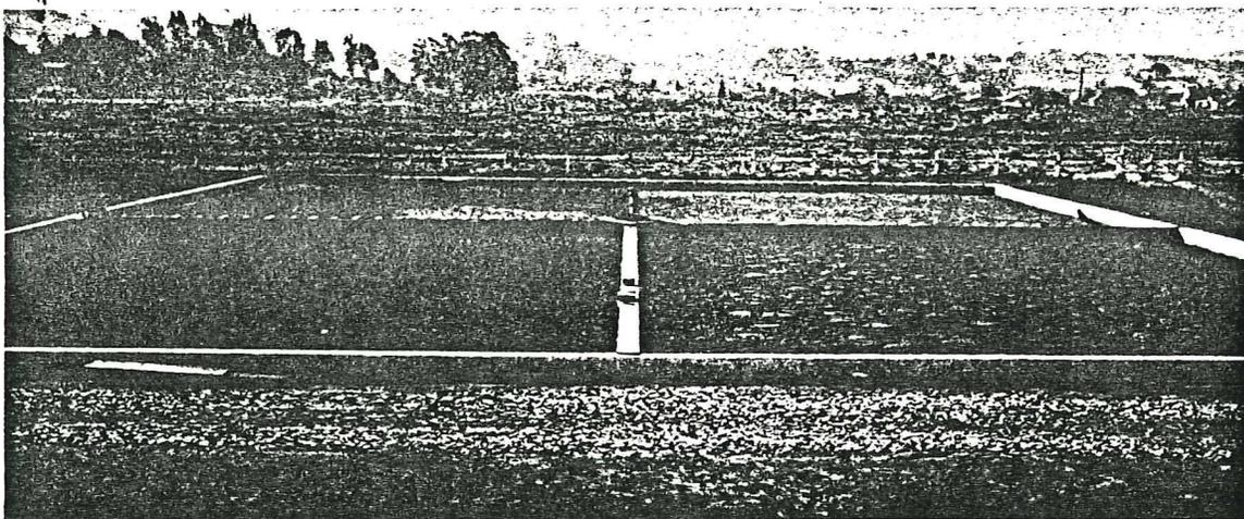
PHOTO 12 - Petaluma Sewage Disposal Plant. Sludge drying beds.
