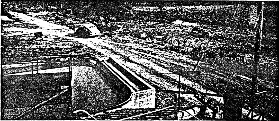
PHOTO 15 - Sebastopol Sewage Disposal Plant showing primary settling tank. Municipal garbage dump in left distance. Channel on right carries effluent from sludge pond Speas Mfg. Co. and, in winter, raw sewage which by-passes Plant during and after storm periods.
