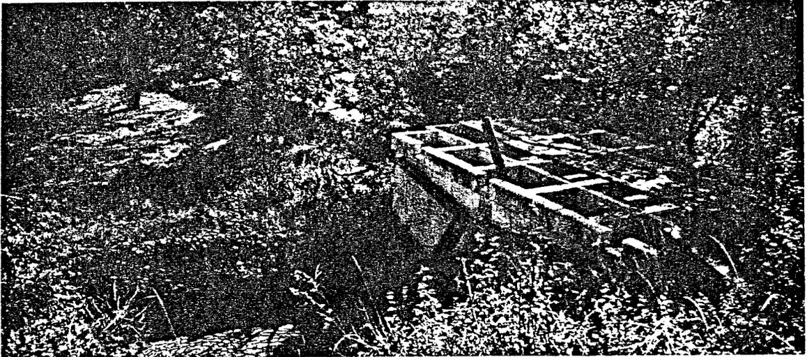
PHOTO 19 - Imhoff tank and sludge drying bed at Cloverdale Sewage Disposal Plant.
