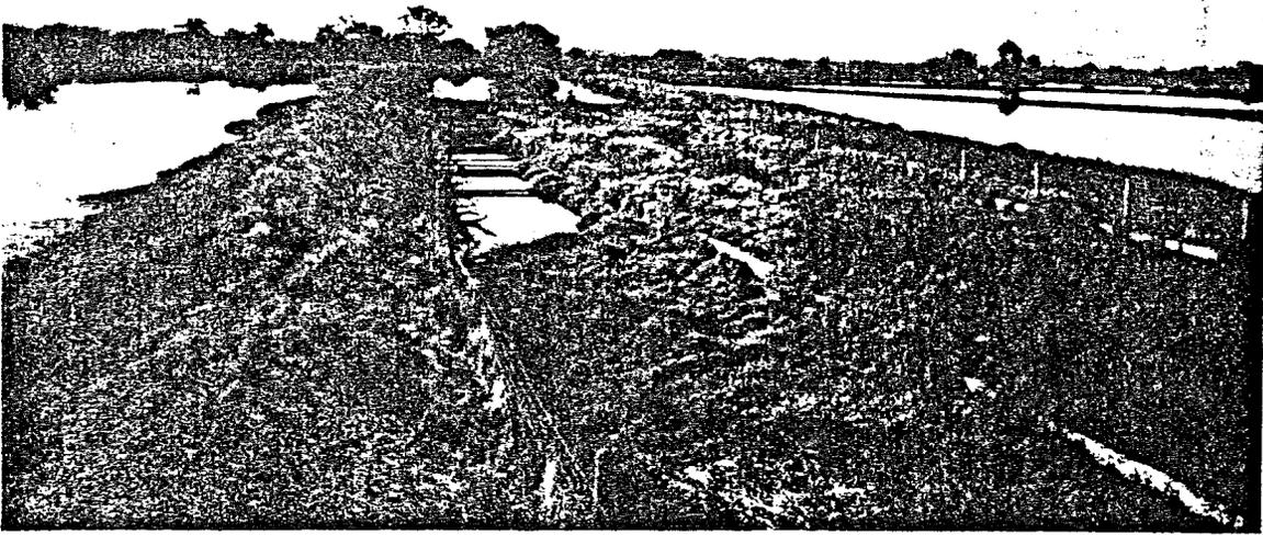
PHOTO 2 - Santa Rosa Sewer Farm showing wooden septic tanks. Two chlorinator houses appear as white square spots in distance.
