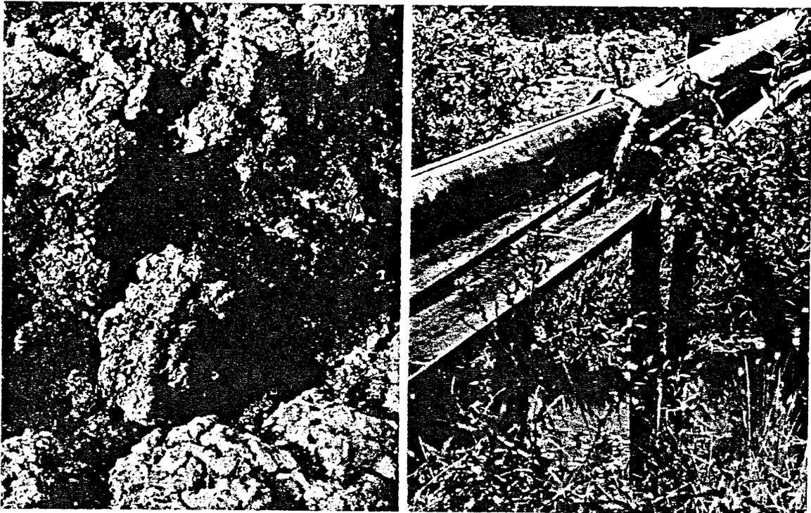
PHOTO 6 - Santa Rosa Sewer Farm close-up of crust on settling tank showing fly larvae in deep crevices.
