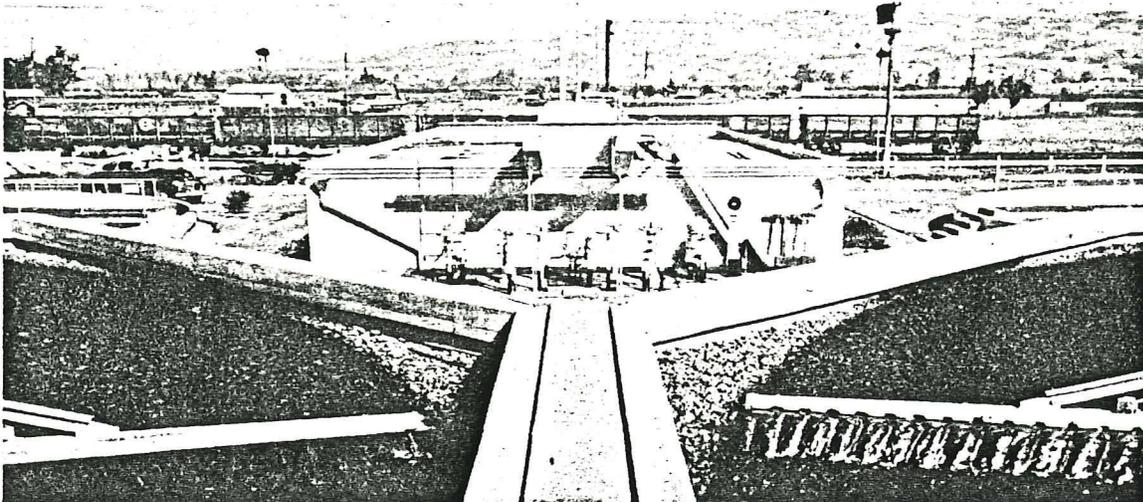
PHOTO 11 - Petaluma Sewage Disposal Plant. Trickling filters in foreground. Administration Building pumps and sludge digestion tank in center and primary and secondary settling tanks on left and right.
