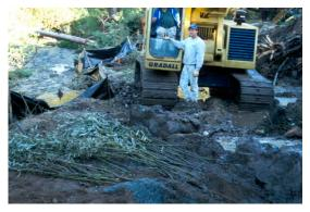
riprap and filter layer to the native soil. Live cuttings can be included and should consist of relatively straight willow branches, 25-40 mm (1-1.5 inches) diameter and long enough to reach beyond the riprap and filter layer and into native ground.
