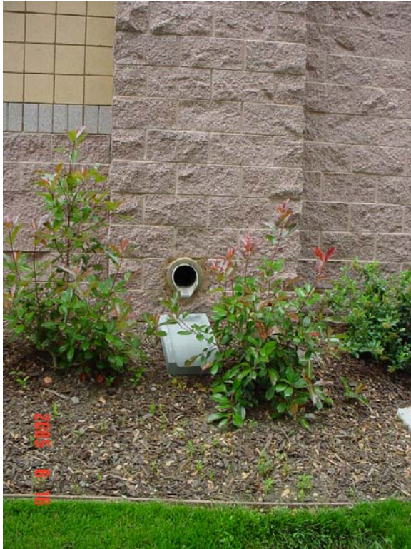
The rooftop runoff drains to the landscaping surrounding the building.
