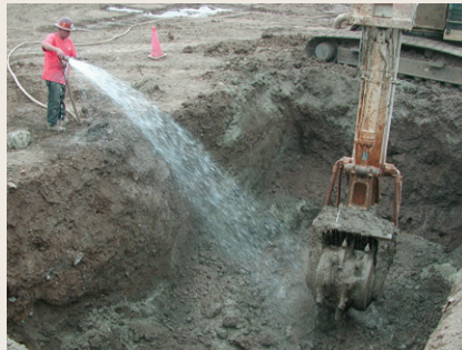
FIGURE 2: SOIL MIXING APPLICATION
