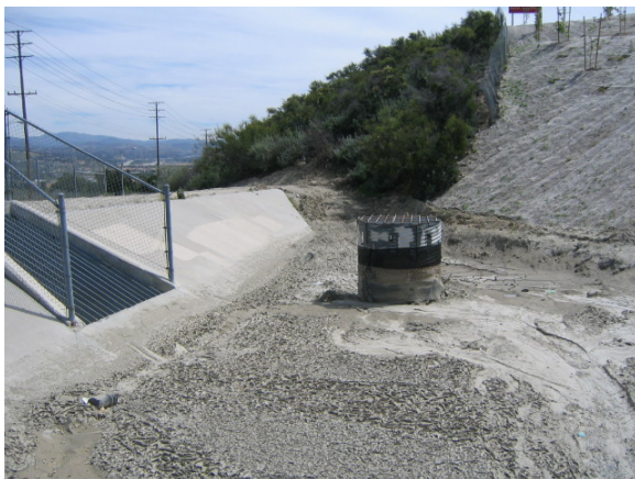
Photo 8: Sediment basin with outlet standpipe.
