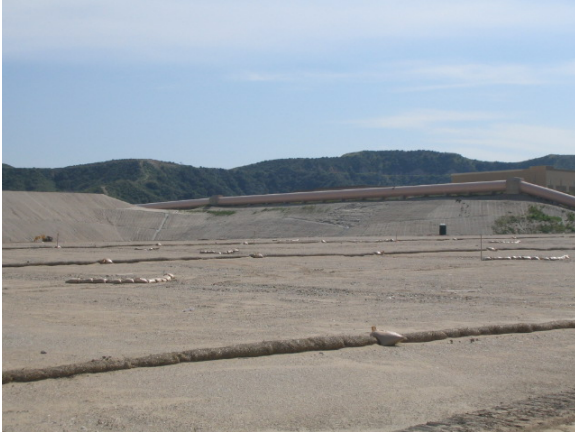
Photo 9. Fiber rolls on flat slope.
