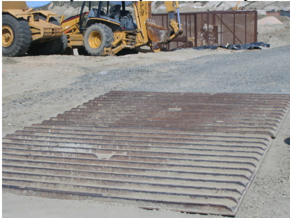
Photo 12. Rumble pads for tracking control.
