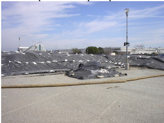
Photo 16. Stockpiles covered with visqueen.
