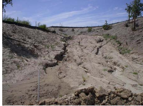
Photo 4. Rills/gullies forming along slope without erosion controls.
