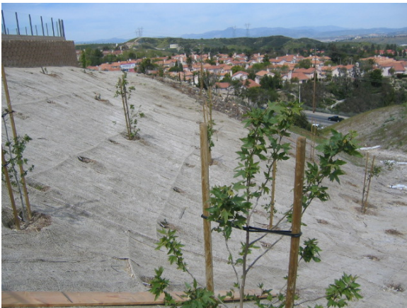
Photo 5. Slope stabilization with jute netting.
