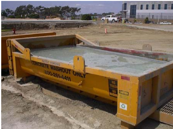
Photo 19: Commercial concrete washout.
