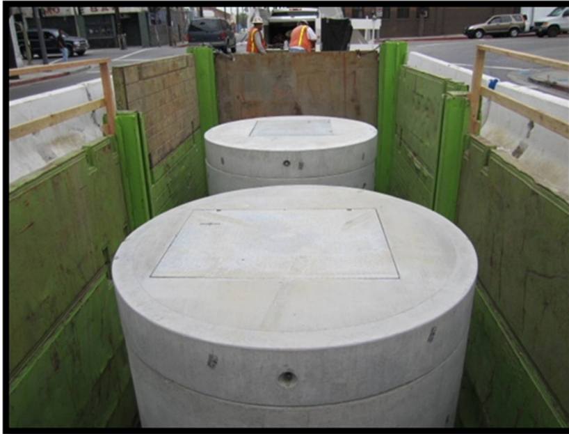
Wet Well and Valve Vault SZW00065
