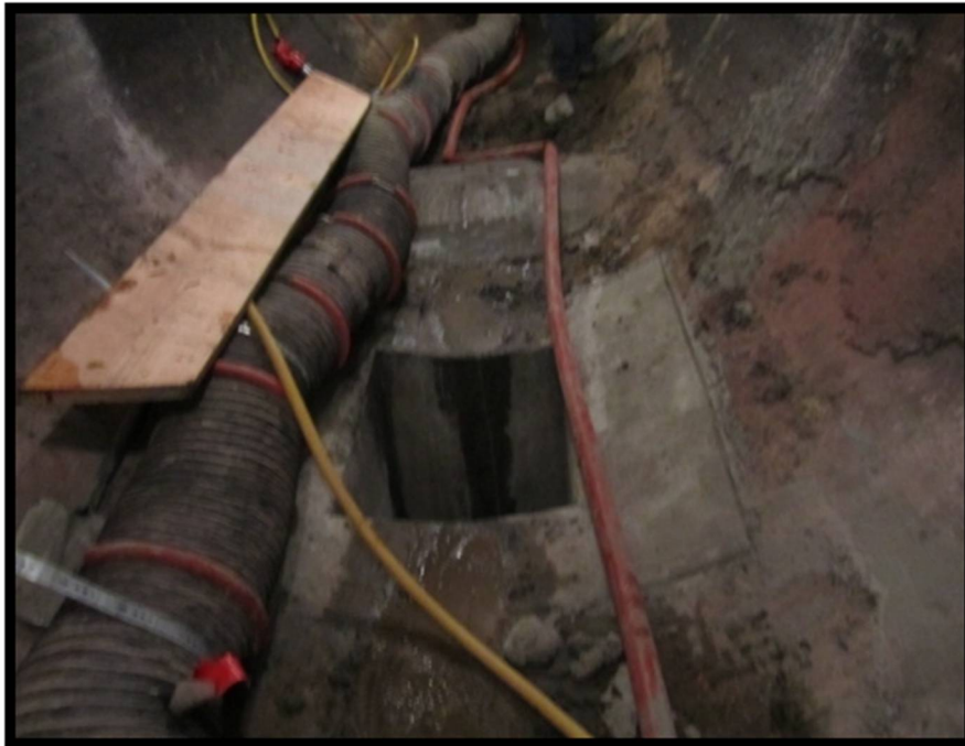
Diversion Opening and Flow Bypassing inside existing SD
