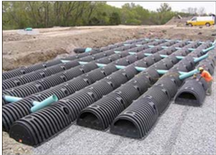
Figure 5-5: Example of StormChamber Units
