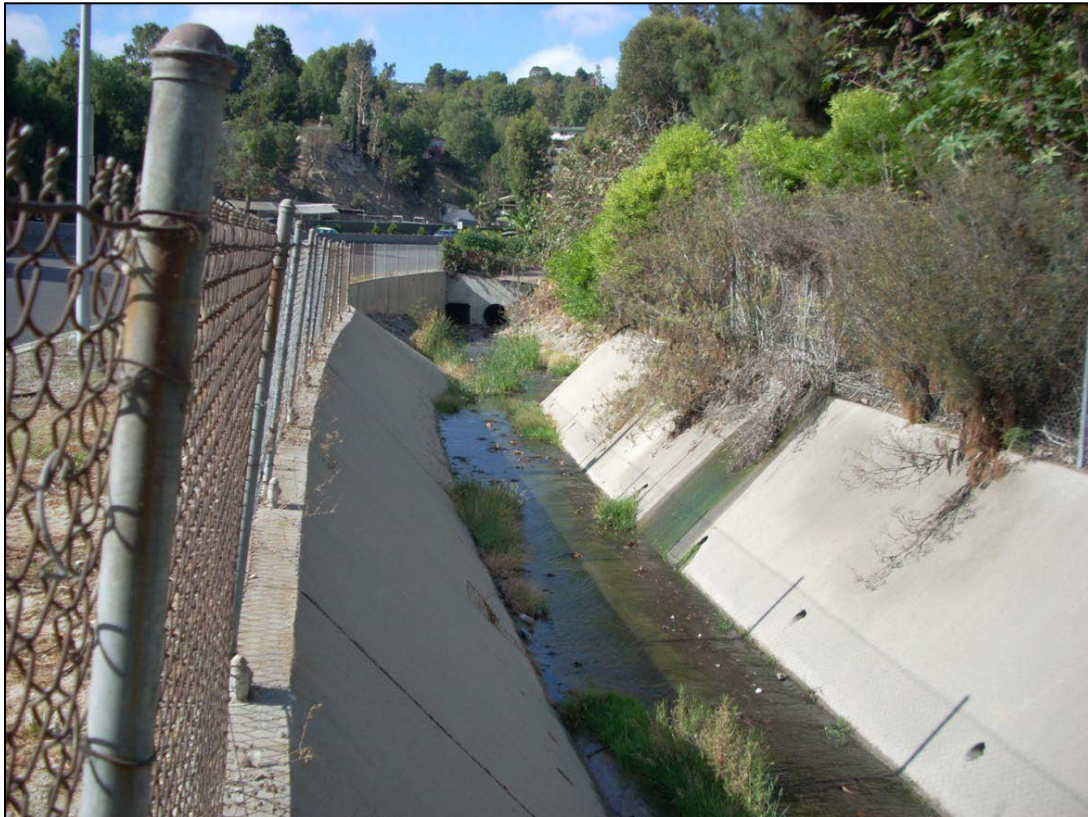
Figure 3-21: RDD 275 – Looking South/Upstream along Crenshaw Boulevard.
