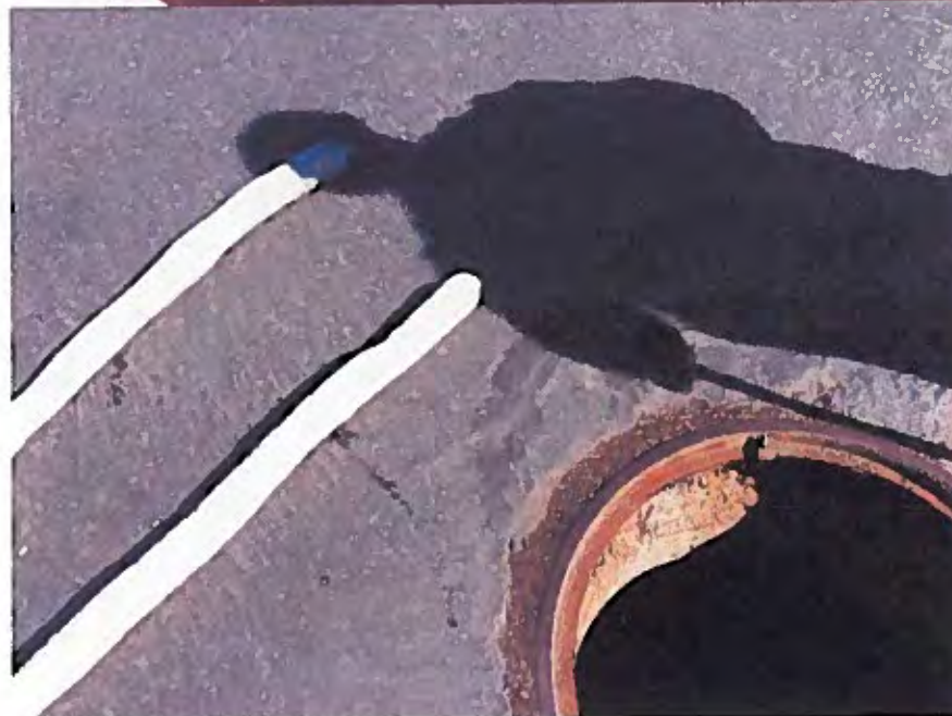
Absorbent boom after placement in storm drain pipe upstream from Ski Run Marina, no oily material present
