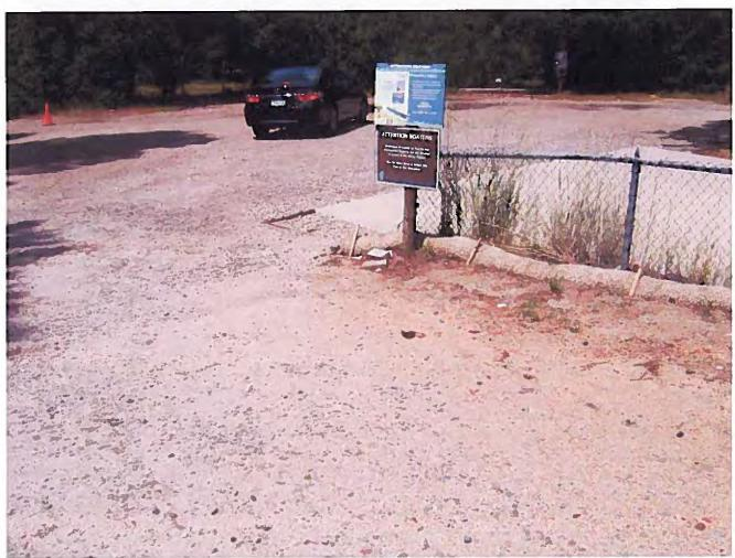
Photograph 04 - Looking East, Northeast at fiber roll. The fiber roll is not J-Hooked at its end which is also installed perpendicular to the grade lower than the rest of the fiber roll, and not parallel to the grade. Any runoff that flows toward the fiber will flow along it toward the downgradient end and, eventually, down the boat ramp and into the marina.
