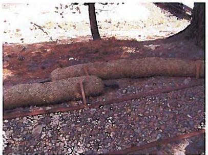
Photograph 19 - West of photo 18, between 3rd and 4th ramps west of office. In this area, the fiber rolls are adequately overlapped.
