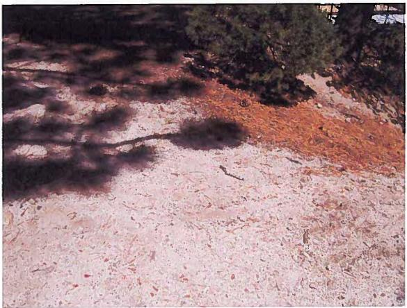
Photograph 26 - 20 feet west of 4th walkway ramp from office, facing east. No fiber roll has been installed, and a small gully erosion can be observed.
