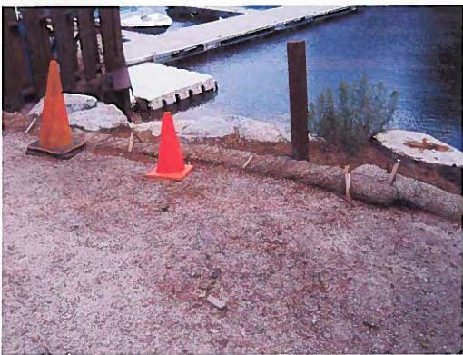
Photograph 06 - BMP joint is not J-hooked, and the fiber roll section by the pylons has been flattened. This area is by marina office, facing southeast
