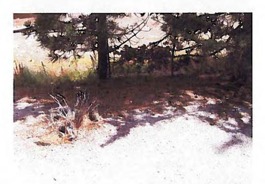
Photograph 29 - Standing at photo point 28, looking southwest. Fiber rolls have not been placed to collect potential stormwater runoff from the unpaved parking area.
