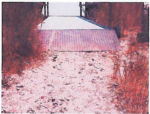
Picture 2: The walkway is downward sloping from the parking lot to the gangways. Potential for rill or guliy erosion into the marina surface waters is possible.
