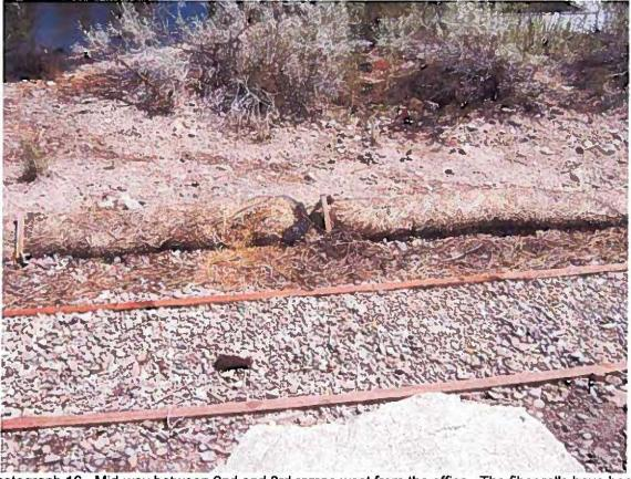
Photograph 16 - Mid-way between 2nd and 3rd ramps west from the office. The fiber rolls have been slightly flattened, and the ends have not been overlapped leaving a gap between the rolls where stormwater runoff can become concentrated.
