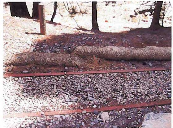
Photograph 18 - Midway between 3rd and 4th ramps west of office. The ends of the fiber rolls are degrading, and they are barely overlapped.
