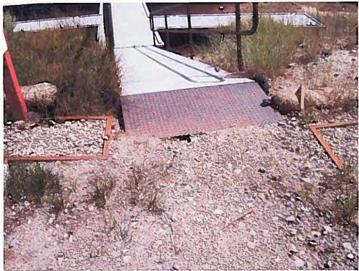
Photograph 17 - 3rd ramp west from office, facing south. A rill has formed beneath the metal plate, creating a threatened discharge of sediments into the marina. No fiber rolls or other BMP exists to prevent runoff from flowing down this area and causing bank erosion.
