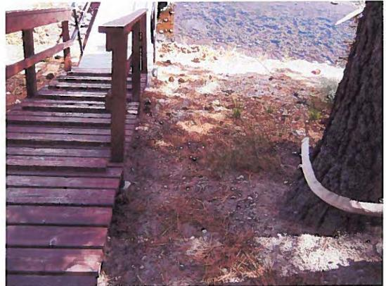
Photograph 24 – Close-up of the west side of the 4<sup>th</sup> walkway shown in Photograph No. 20. Evidence of erosion can be observed.
