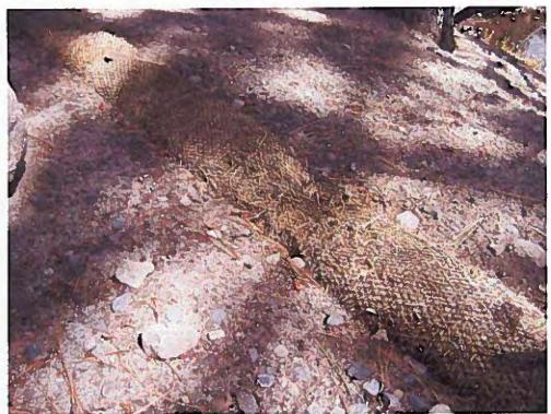
Photograph 25 - 10 feet west of the 4<sup>th</sup> walkway west of the office. The fiber roll has degraded.
