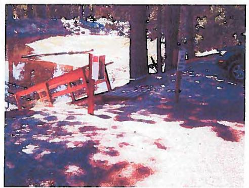
Picture 3: Gangway number three is also in a low depression of the hillside. These are potential sediment sources as there are no BMPs installed.
