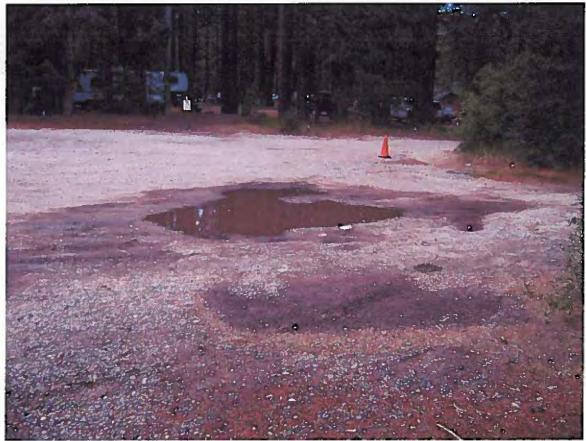
Photograph 02 - Facing West Towar Parking Area, Panning right of Photo 1, Standing Ponded Water in Lot From Recent Rains
