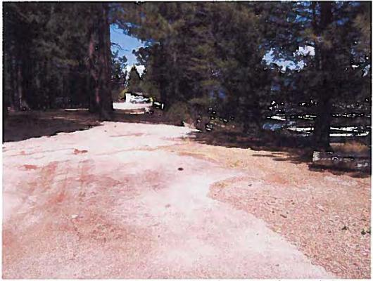
Photograph 32 - At west end of the marina boundary in the boat trailer parking area looking east. Fiber rolls were not installed at trailer parking area. Note the evidence of ponded water in the middle of the photograph, indicating fiber rolls may not be necessary in this area.
