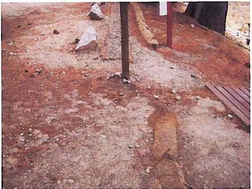
Photograph 23 - Close up of the sediment-inundated fiber roll shown in Photograph No. 20, facing east. The fiber roll end in the foreground was slightly J-Hooked to capture runoff and sediment, while the end of the fiber roll at the top of the photograph is not J-Hooked and allows runoff to flow down the embankment. Photograph taken by Will Chen.
