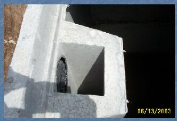
One manufacturer of septic tanks also sells these as grease interceptors. This is a concrete effluent baffle wall. The problem is that the baffle only extends down 13"...so only approximately 8" will be below the wastewater surface. SHORT CIRCUIT=FOG
