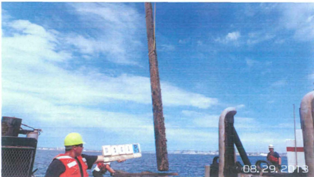
Concrete pier pilings removed from the A-8 Anchorage
