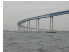
San Diego Bay bridge
