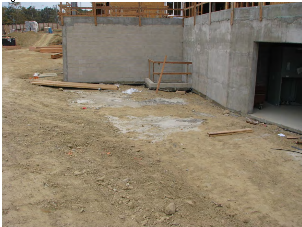
Figure 14. Concrete washout with no containment
