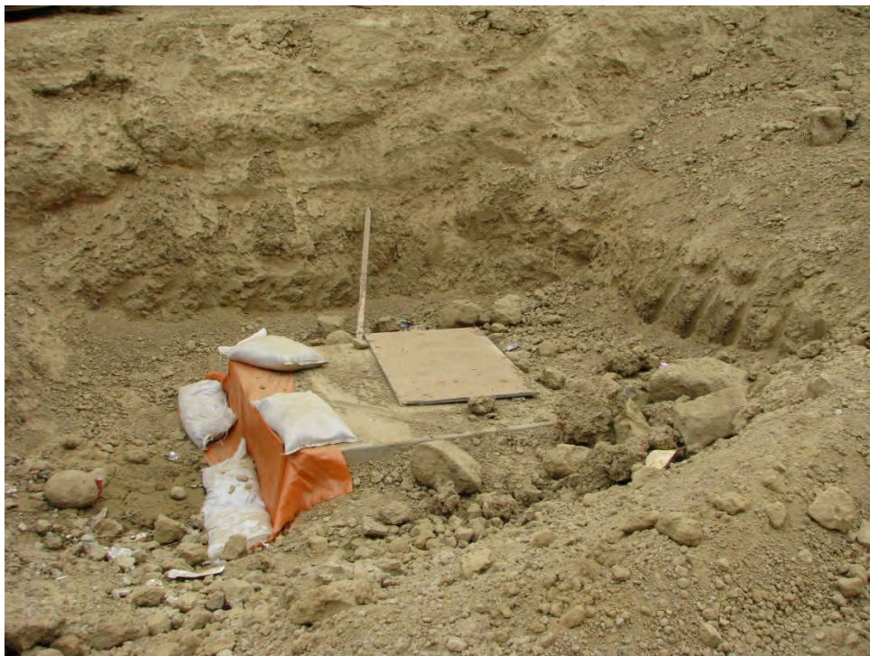
Figure 20. Live storm drain covered with permeable fabric
