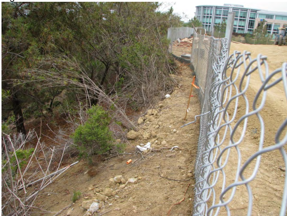
Figure 12. Sediment discharge outside site boundary
