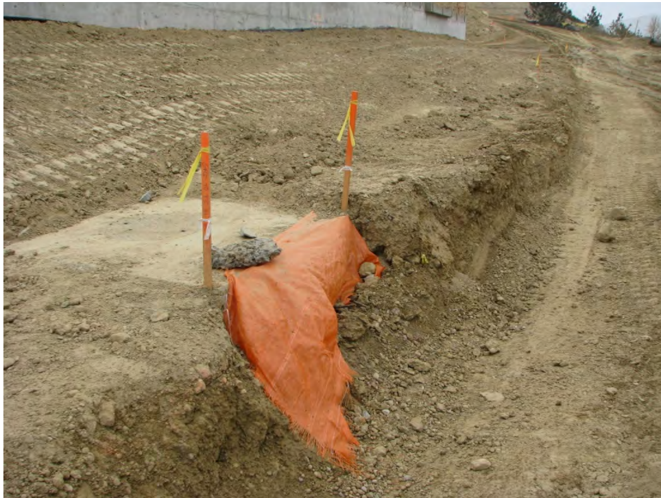
Figure 19. Live storm drain covered with permeable fabric
