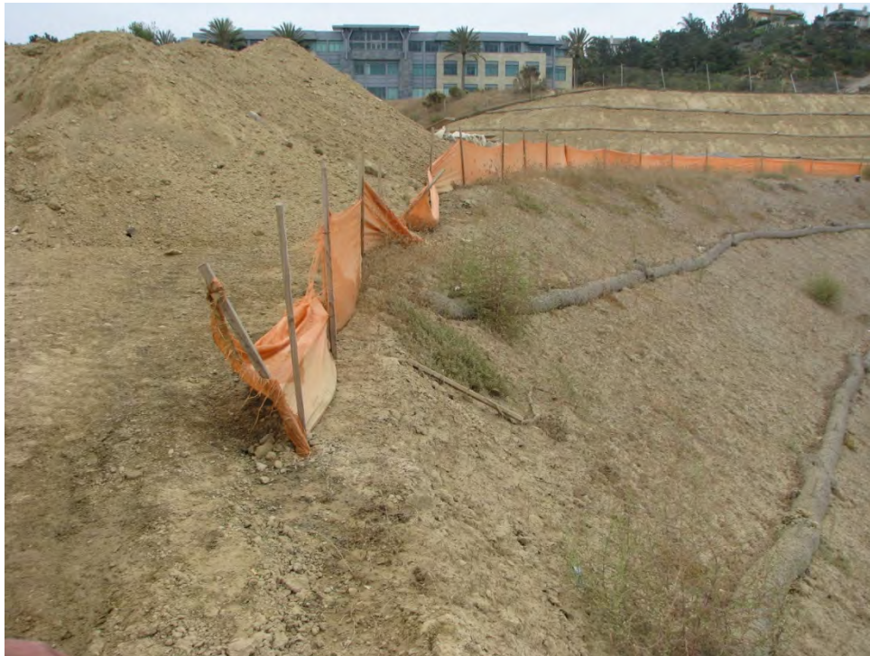
Figure 9. Sediment stockpile with broken silt fence
