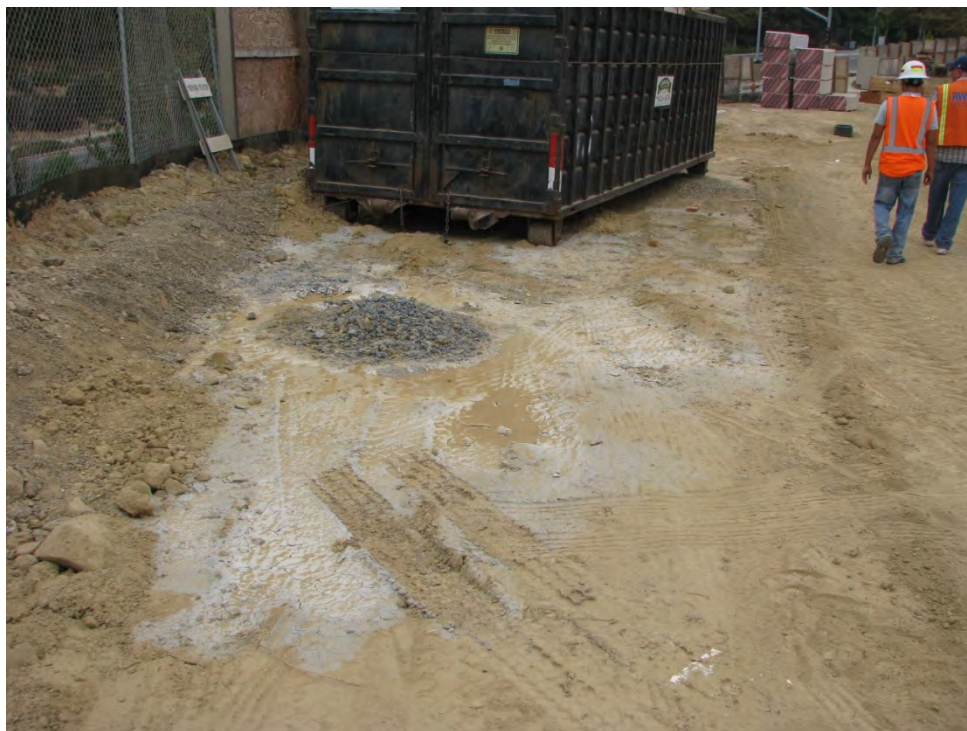
Figure 13. Concrete washout with no containment
