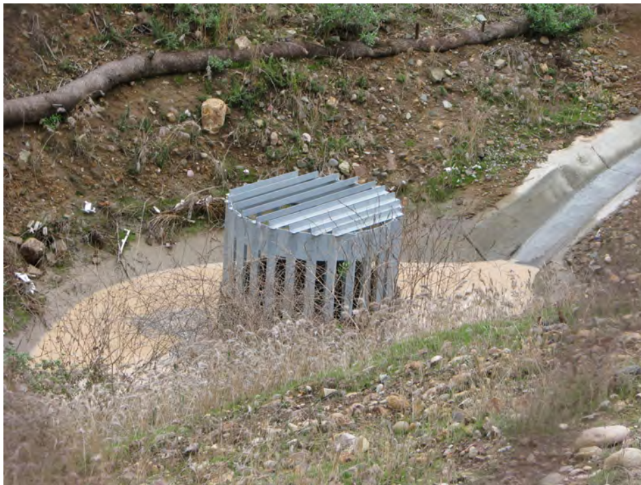
Figure 8. Storm drain on Caltrans right of way (East side project boundary)
