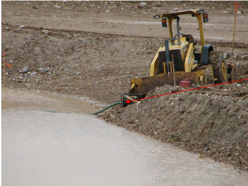
Figure 11. Pump intake
