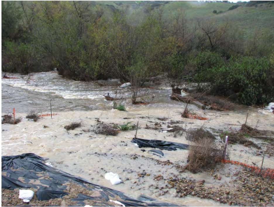
Figure 9. Construction site discharge entering Lusardi Creek
