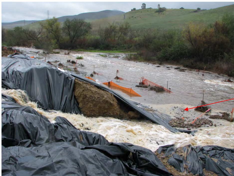
Figure 8. Construction site discharge entering Lusardi Creek
