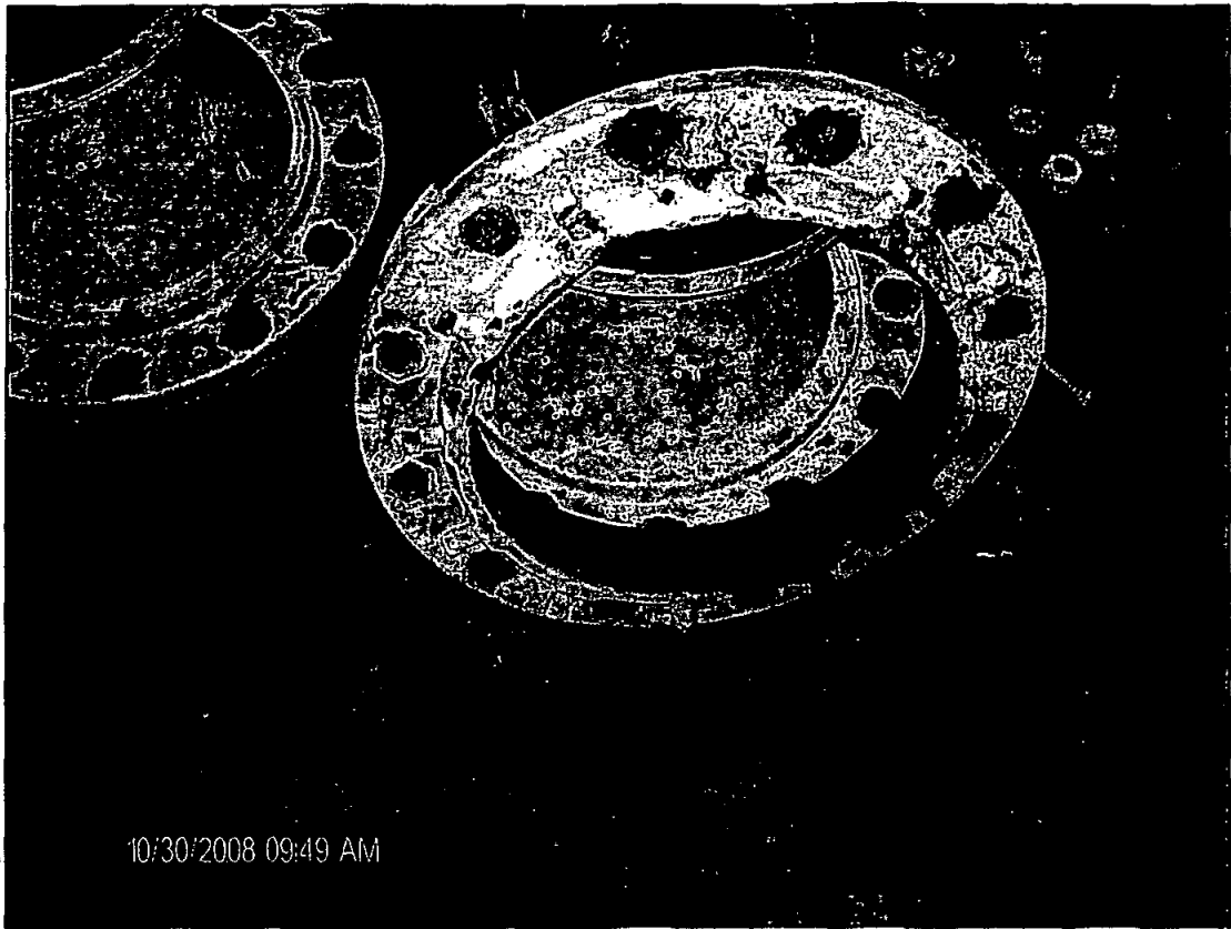
Photo #13: Pump #1 Uni-Flange Coupling
