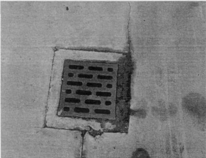
Photo 3 Loading dock storm drain showing pellets around and in the storm drain
