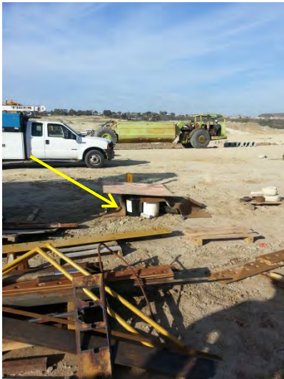
Photo 3: Chemicals were not stored in watertight container or storage shed. Waste without secondary containment and not protected from wind and rain.
