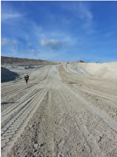
Photo 9: No erosion controls present on large slopes. No linear sediment controls on large slopes. No erosion in conjunction with sediment controls present on other areas of site.
