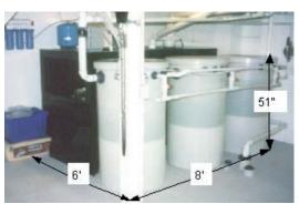
**Figure 2-8** The Equaris greywater treatment system. (Adapted from Equaris, Inc.)
