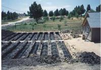
Figure 11-21 Installation of Infiltrator chamber systems. (Adapted from Infiltrator Systems Inc.)
