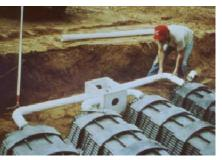
**Figure 11-14** Installation of the Biodiffuser chamber system. (Adapted from ADS, Inc.)
