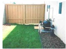
**Figure 2-7** The ReWater filtration system and irrigated landscape. (Adapted from ReWater Sys Inc.)
