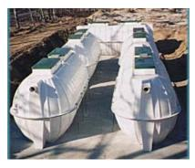
**Figure 7-14** Cromaglass treatment system using multiple units anchored to concrete pad to prevent flotation. (Adapted from Cromaglass Co.)
