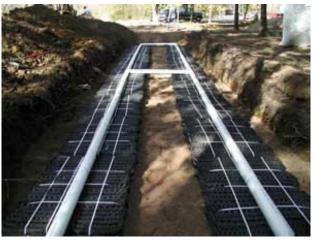
**Figure 11-20** The In-Drains system for the treatment and infiltration of wastewater. (Adapted from Eljen Corporation)
