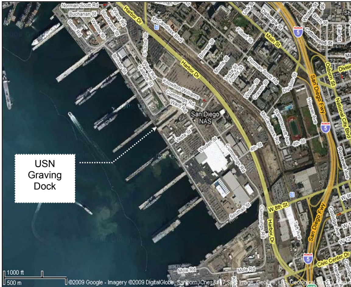
Figure B-9. USN Graving Dock at NBSD
