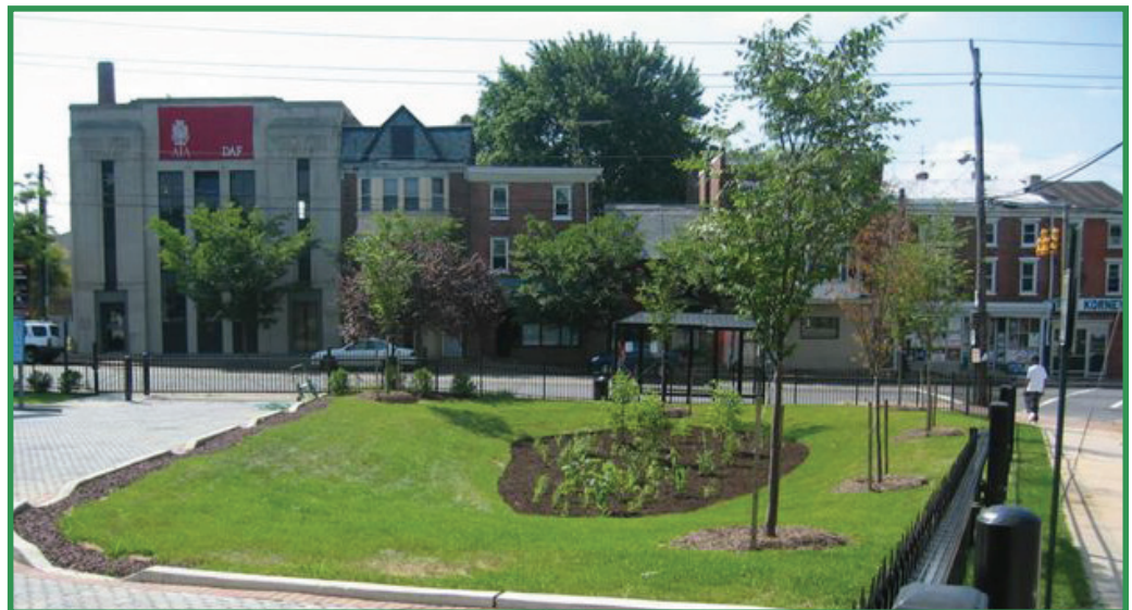
A bioswale in Wilmington, Delaware, designed to absorb and retain stormwater runoff.
